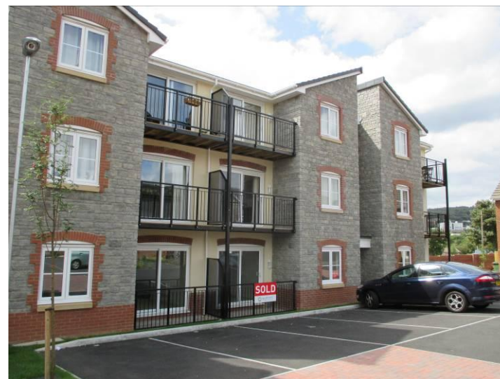
Car parking areas should be well overlooked
