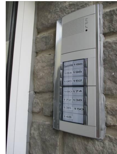
Communal entrance intercom
