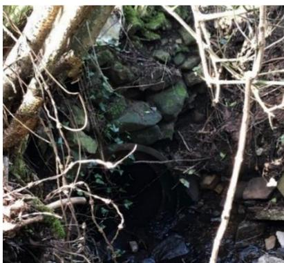
**Photograph 40:** Stone walls associated with the eastern entrance of Culvert 3 (note Building 15 located on top)
