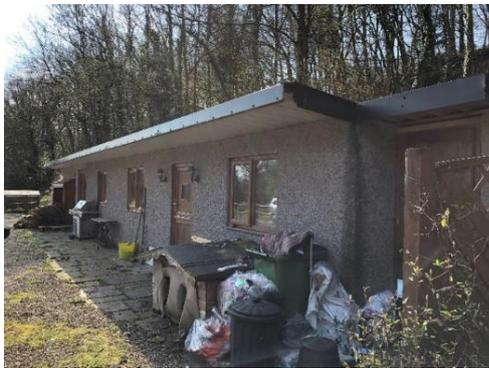
Building 11B was a stable building to the north the Signalman’s Cottage. It was a block-built, single skin, one-storey building with a steel-sheet roof. The building was assessed as having a negligible potential for roosting bats.
