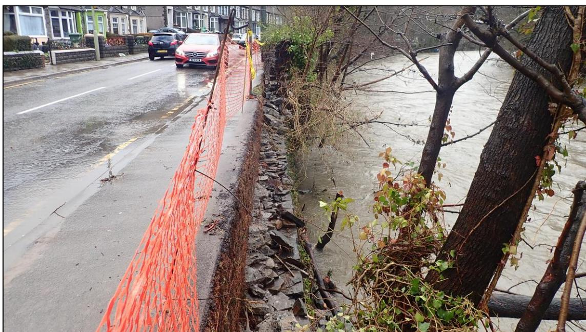
**Figure 5:** Collapsed river wall (NFD) on Berw Road following Storm Dennis (captured by RCT's Flood Risk Management team on 17<sup>th</sup> February 2020)
