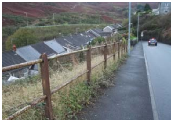
Photograph 6: Barrier at Rd Leading to Aberllechau Road
