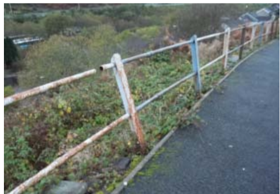
Photograph 7: Damage to Barrier
