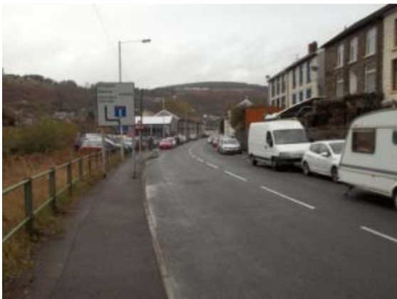
Photograph 3: Margaret Street O/S No. 40 Looking West
