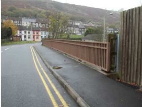
Photograph 11: Guardrail at Railway Bridge
