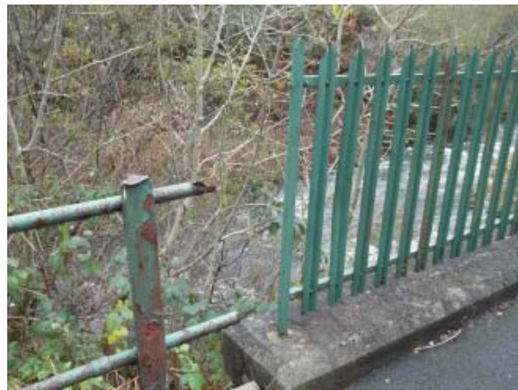
Photograph 10: Damage where Guardrail Meets Fence on Aberllechau Road
