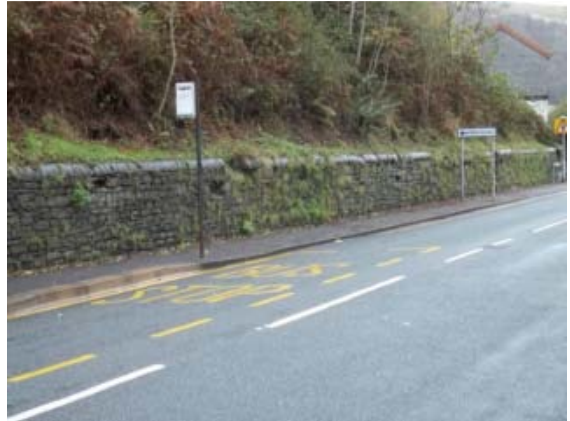
Photograph 12: Retaining Wall on Aberllechau Road
