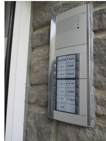
Communal entrance intercom
