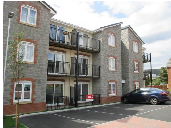
Car parking areas should be well overlooked
