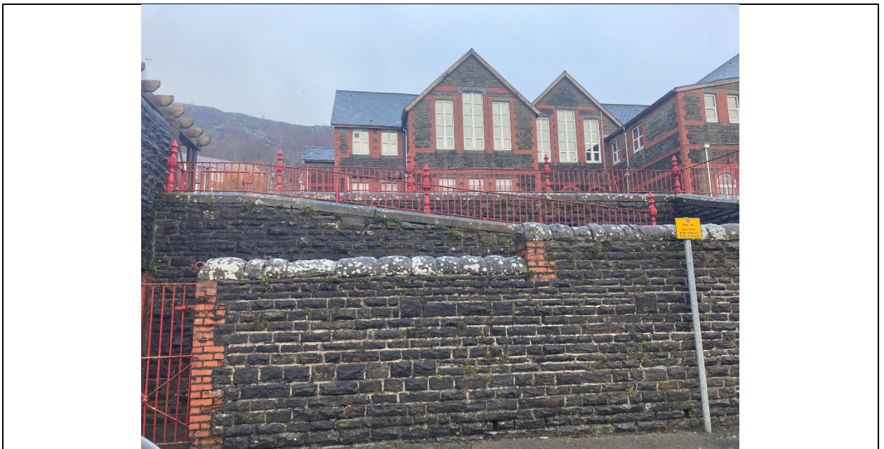
The view of the existing school building from Darran Terrace.
