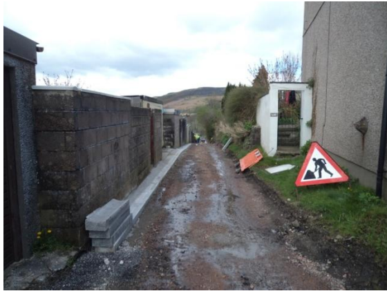
Photo 6 – Lane during Construction.
