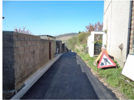
Photo 7 – Lane After Construction
