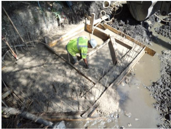
Photo 8 – Headwall Construction
