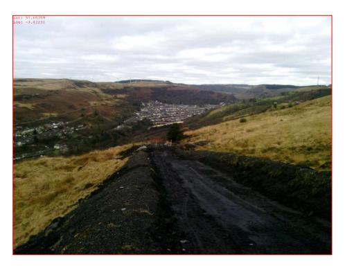
Figure 3.6 Footpath below Llanwonno Upper Tip acting as drainage.
