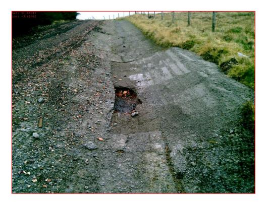
Figure 3.11 Upper sections of Channel 2. Concrete channel with visible damage.
