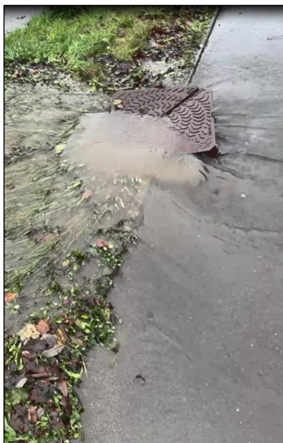
Figure 6: Surcharging manhole at Coedcae Road ('Manhole 1') (image captured by a local resident).
