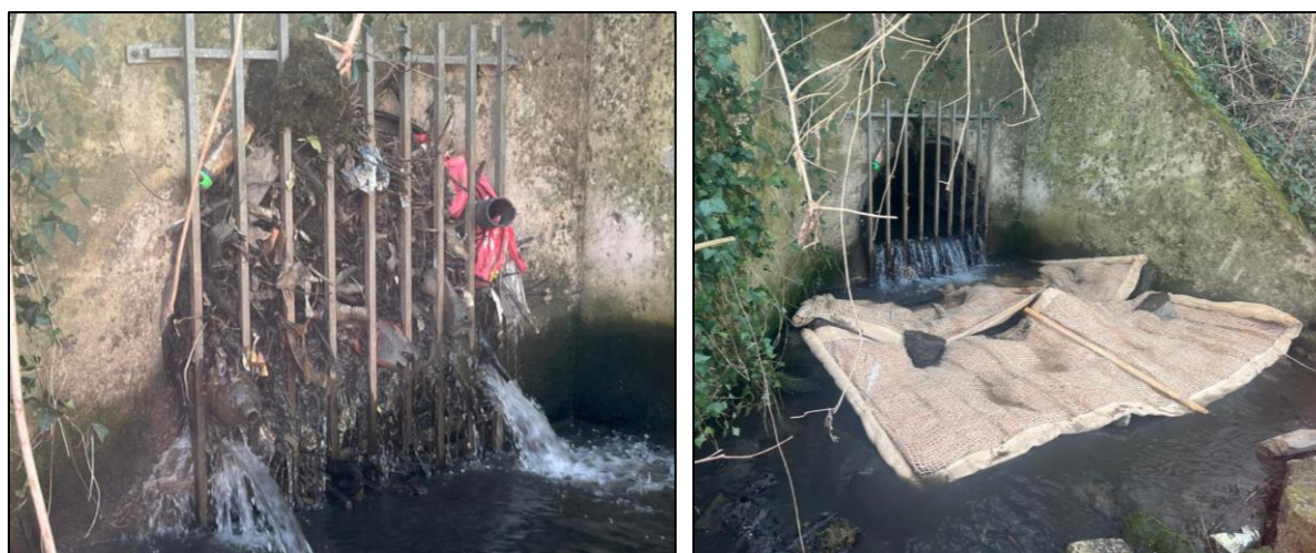
Figure 8: (Left) Significant debris accumulation at the culvert out post event. (Right) Culvert outlet post cleansing utilising appropriate silt control measures (images captured by RCT's FRM team post event).
