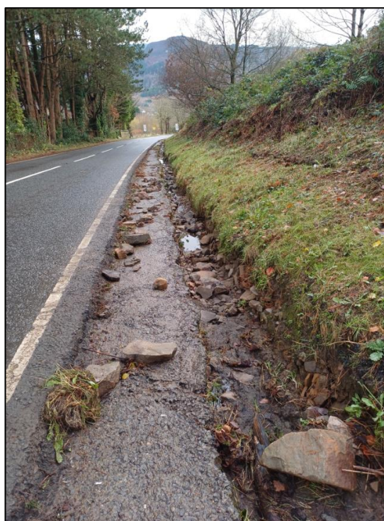
Figure 9: Evidence of scoring to the highway verge as a result of mobilised debris during the storm event (captured by RCT's Flood Risk Management team on 27 November 2024).
