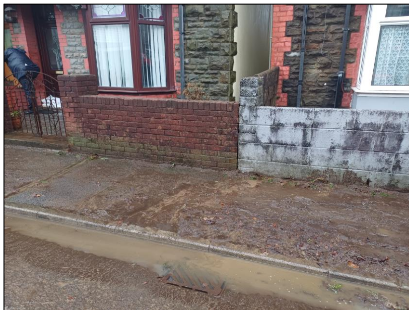
Figure 21: Evidence of silt deposited and blocked highway gullies along Hill Street (captured by RCT's Flood Risk Management officers on 24/11/2024).
