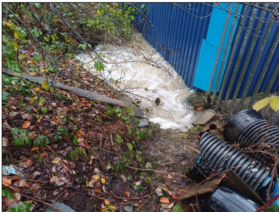
Figure 4: Evidence of submerged 'Culvert Inlet 1' which surcharged during Storm Bert (captured by RCT's FRM team on 24 November 2024).
