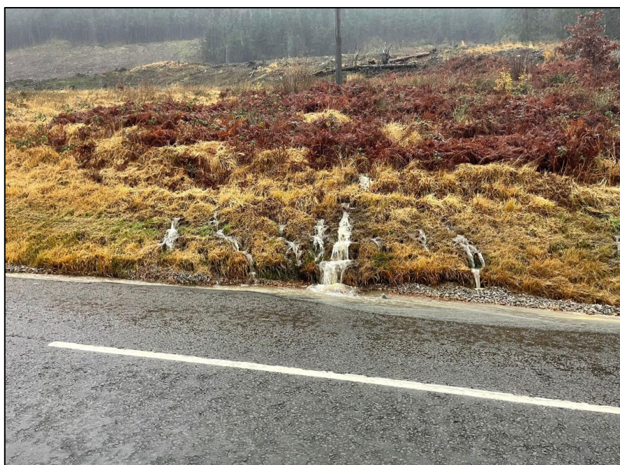
Figure 10: Surface water flows conveying overland from the steep area of hillside above Rhigos Road (image captured by a Council officer at 15:00 24 November 2024).
