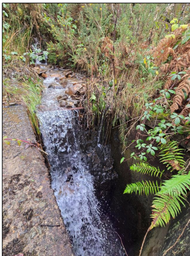
Figure 14: Evidence of blockage caused by stonewash to the upper debris screen associated to 'Culvert Inlet 3' (captured by RCT's Flood Risk Management team on 27 November 2024).
