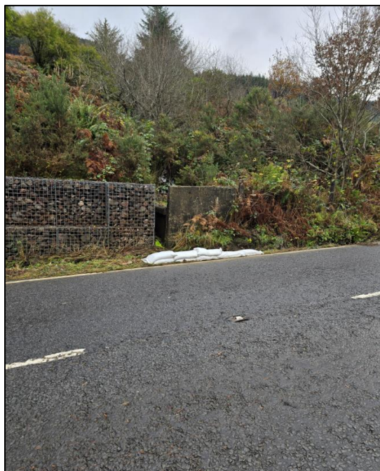
Figure 8: Evidence of flattened grass and sandbags to redirect flow at 'Culvert Inlet 3' (left) and stonewash debris in the surrounding area of 'Culvert Inlet 4' (captured by RCT's Flood Risk Management team on 27 November 2024).
