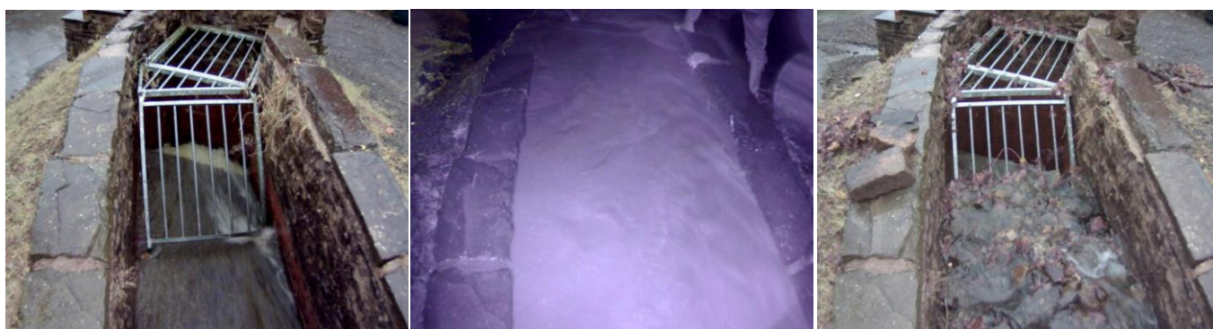
Figure 20: Image of a private culvert inlet in Treorchy pre (left), during (middle) and post Storm Bert (right) showing evidence of overtopping during the event and mobilised debris obstructing the trash screen immediately following the event.
