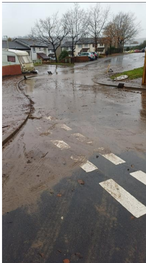
Figure 33: Scour damage to the highway in Beddau (left) and silt and debris deposited along the highway at Rhydyfelin following Storm Bert
