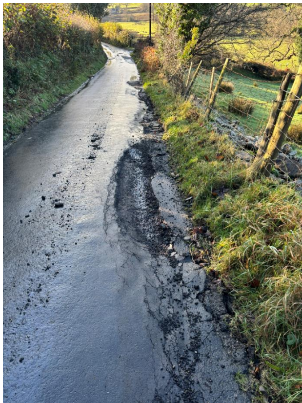
Figure 33: Scour damage to the highway in Beddau (left) and silt and debris deposited along the highway at Rhydyfelin following Storm Bert
