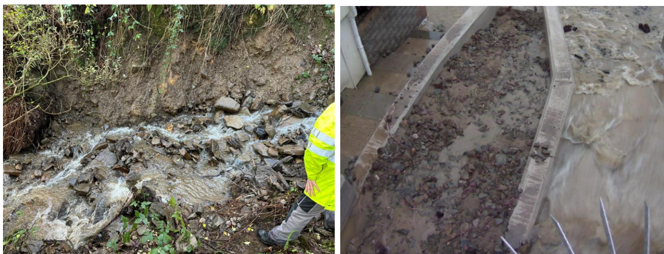
Figure 23: Evidence of scour to the banking of the unnamed ordinary watercourse (left) and the subsequent deposition of material downstream at the Heath Terrace Central culvert inlet in Ynyshir (right) during Storm Bert.
