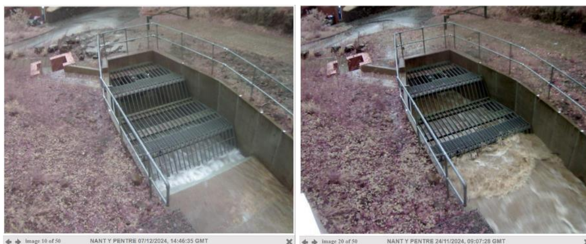
Figure 30: The response of the Pentre Road culvert inlet improvements in Pentre during the peak of Storm Bert
