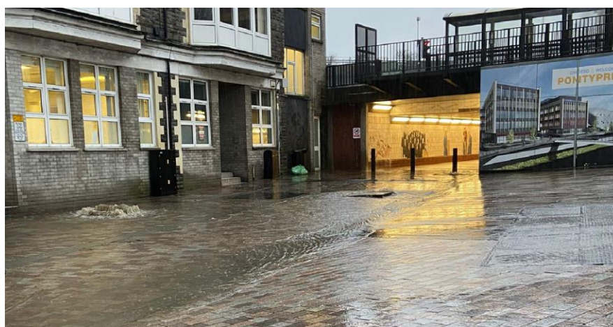
Figure 28: Two combined sewer manholes showing evidence of surcharge at Mill Street, Pontypridd during Storm Bert
