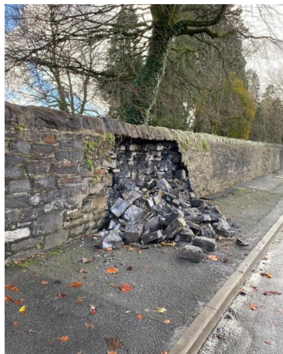
Figure 31: Landslip at Tylorstown in the Rhondda Fach (left) and collapsed retaining wall at Aberdare Park (right) captured following Storm Bert
