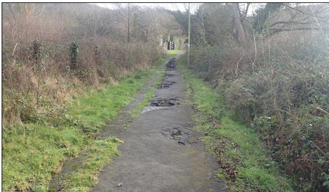
**Figure 11:** Evidence of damages to the top of the path looking up towards Heol Nant (captured by FRM officers on 17<sup>th</sup> February 2020)
