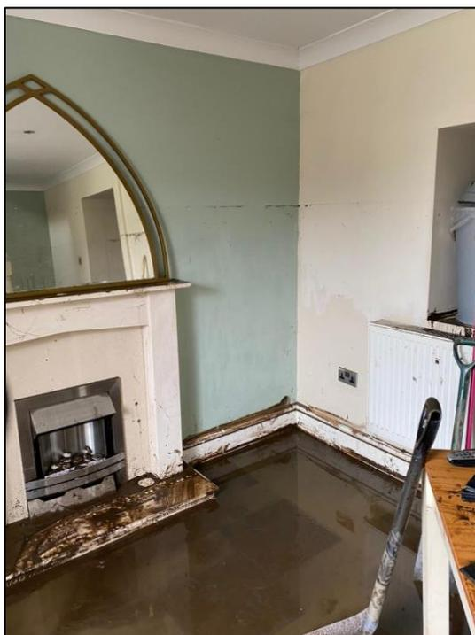
**Figure 7:** Water depth marks in a property at Cilfynydd Road following Storm Dennis (image provided by resident)
