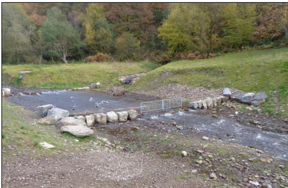
**Figure 24:** Initial upstream debris screen in the Nant Cae Dudwg watercourse captured prior to Storm Dennis
