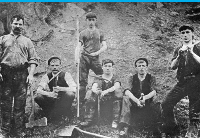
Blaencwm Railway Tunnel Workmen, circa 1885-90
