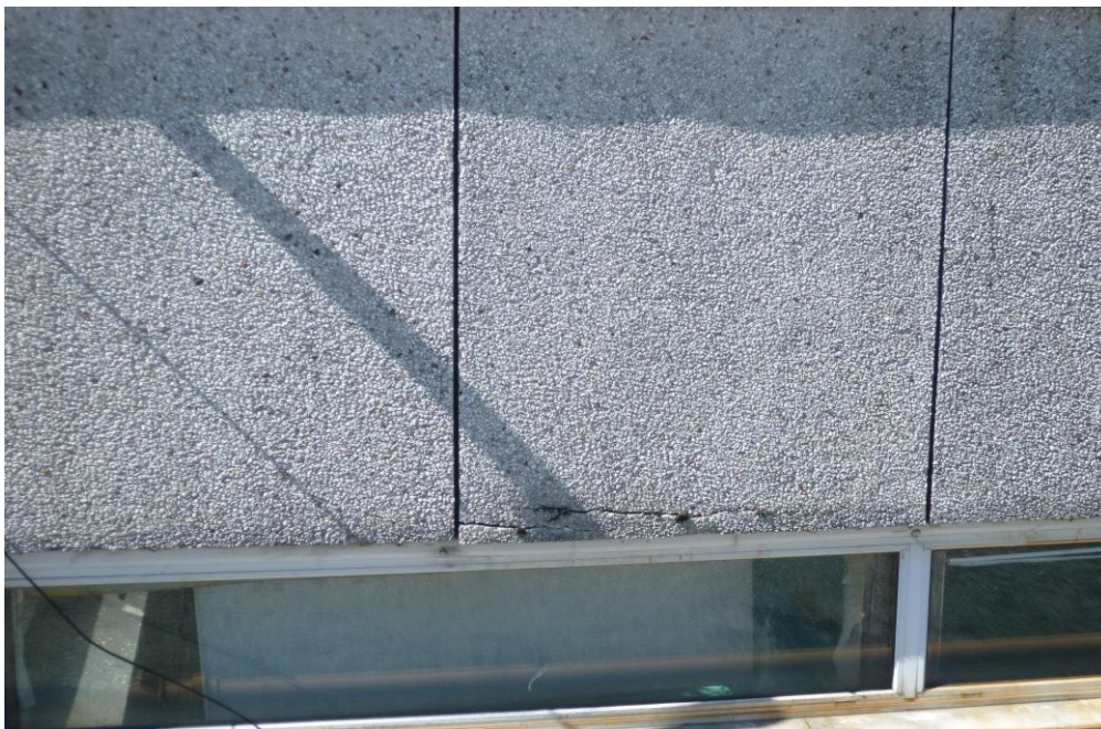
Photograph 4 – External concrete wall panel displaying spalling concrete resulting from corrosion to steel reinforcement bars.
