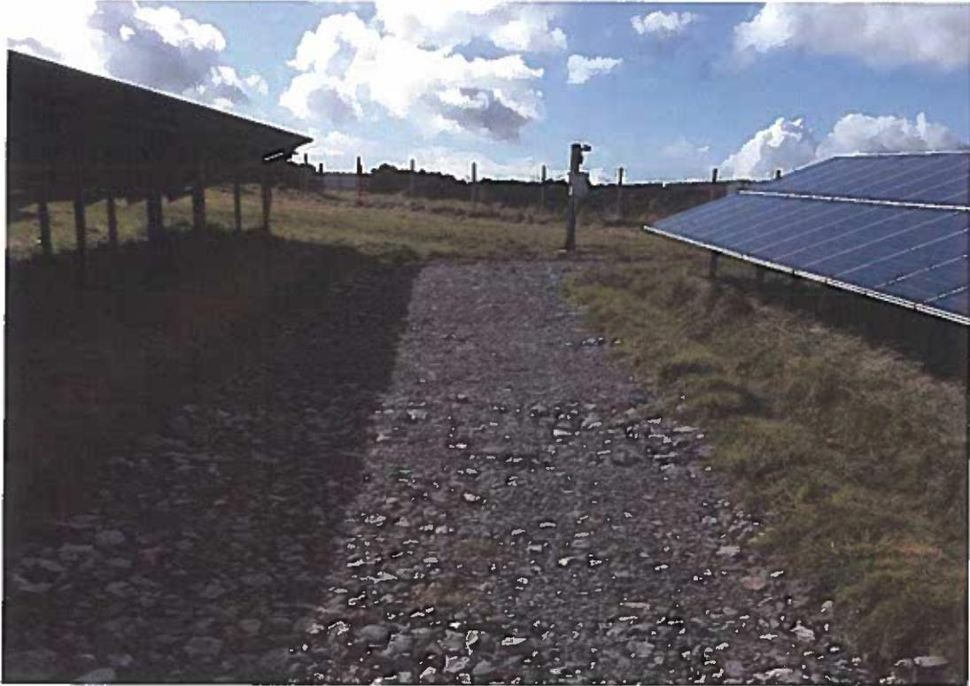
*Figure 3: Close up of access track to illustrate permeability*
