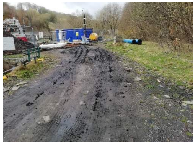
Figure 25 – approach to works site and small footbridge
