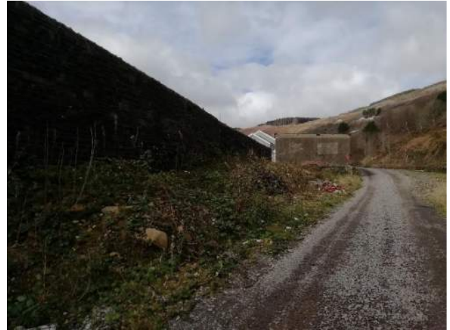
Figure 21 – view northwards from bridge
