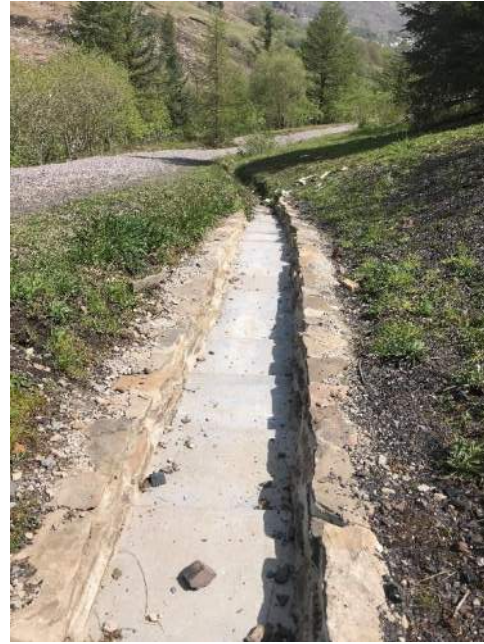
Figure 33 – new concrete drainage
