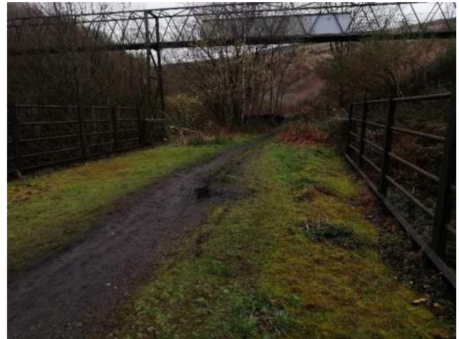
Figure 9 – path running over bridge to east bank of river
