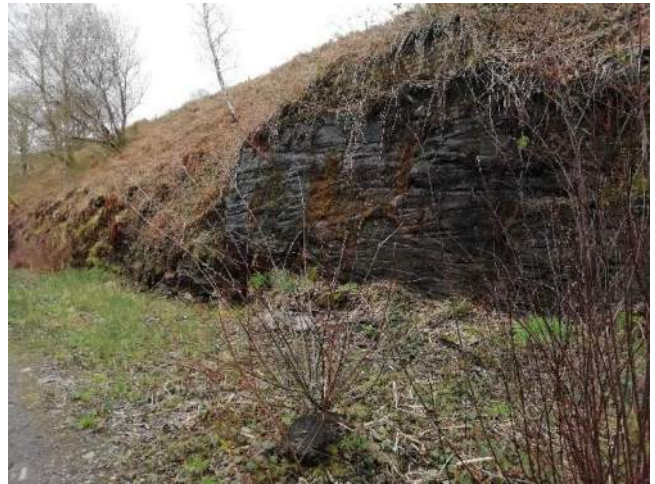
Figure 15 – exposed stone/cliff face on eastern edge of site
