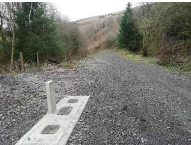
Figure 12 – new concreted structure in path
