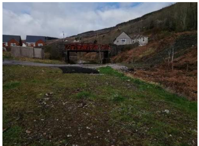
Figure 19 – approaching road bridge
