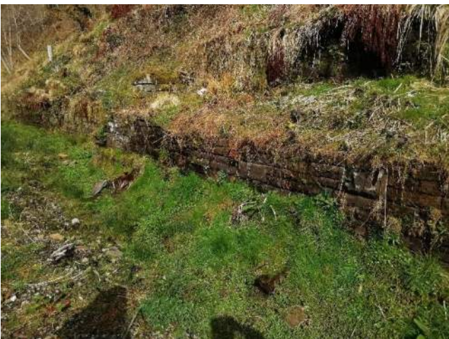
Figure 22 – wall and habitat adjacent (east) to bridge
