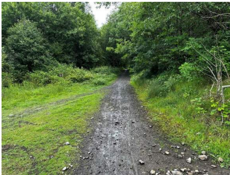
Figure 4 – Photograph of northern end of scheme showing approach to new Blaenllechau North Bridge
