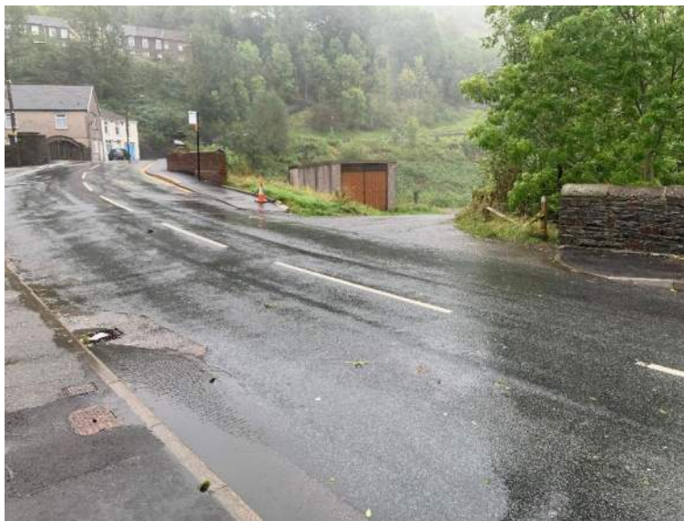
Figure 14 – Station Road, Blaenllechau
