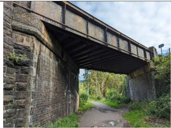
Figure 28 - Road bridge at entrance at south entrance to Phase 5.
