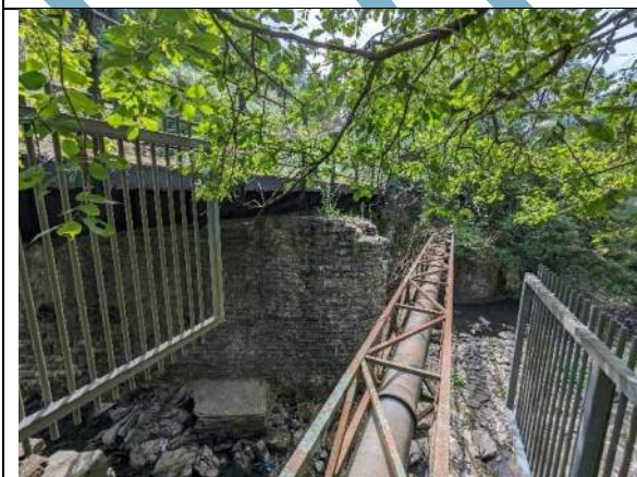
Figure 25 - Tylerstown south bridge.
