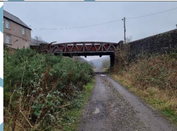
Figure 12 - Bridge at Blaenllechau (not subject to works).
