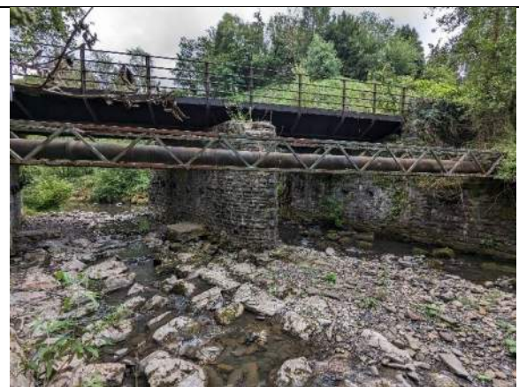
Figure 26 - Tylerstown south bridge.
