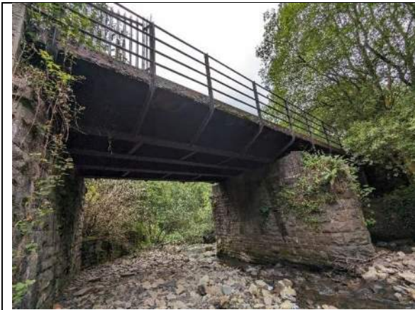
Figure 21 - Tylerstown north bridge.
