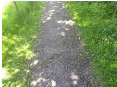
**Photograph 56 – Damage caused to footpath by roots of Tree T70.**
