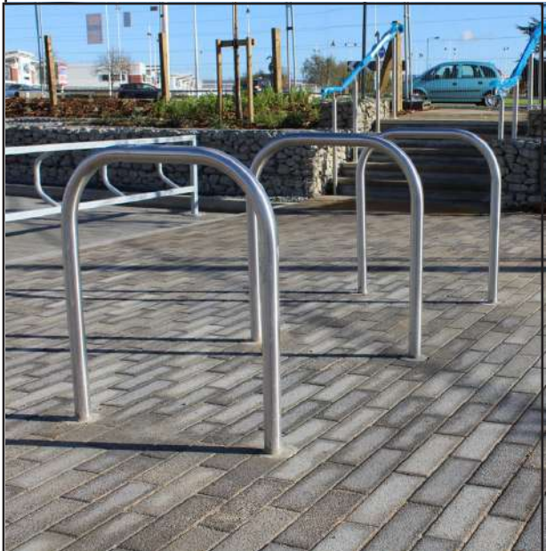
Sheffield bicycle racks bedded in concrete footings
