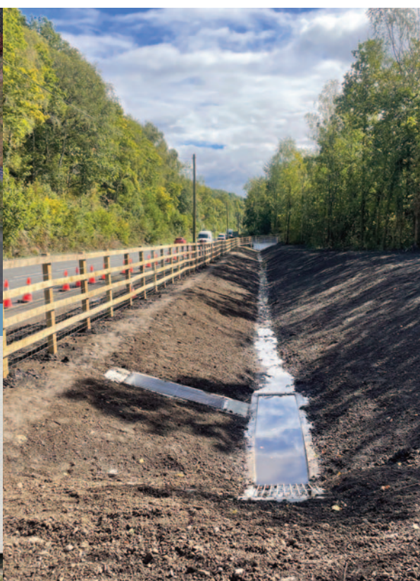
Highway Drainage Swale – A4058, Newtown
