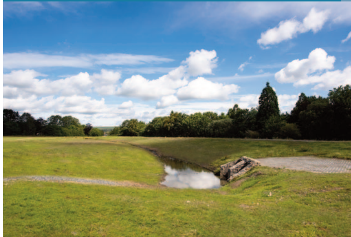
Attenuation Basin - Park Lane Flood Alleviation Scheme, Aberdare
