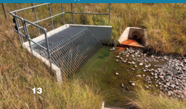
Culvert Inlet Improvement – A465 Rhigos Road
