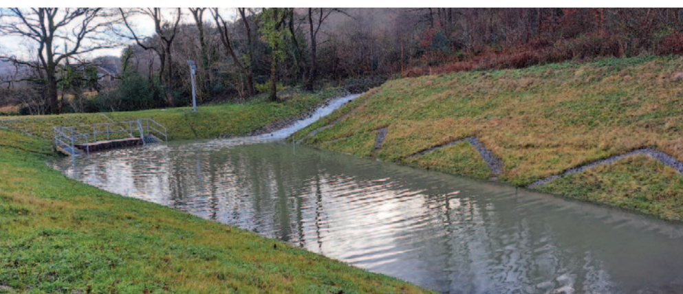
Attenuation Basin – Upper Bronallt Terrace Flood Alleviation Scheme, Abercwmboi
