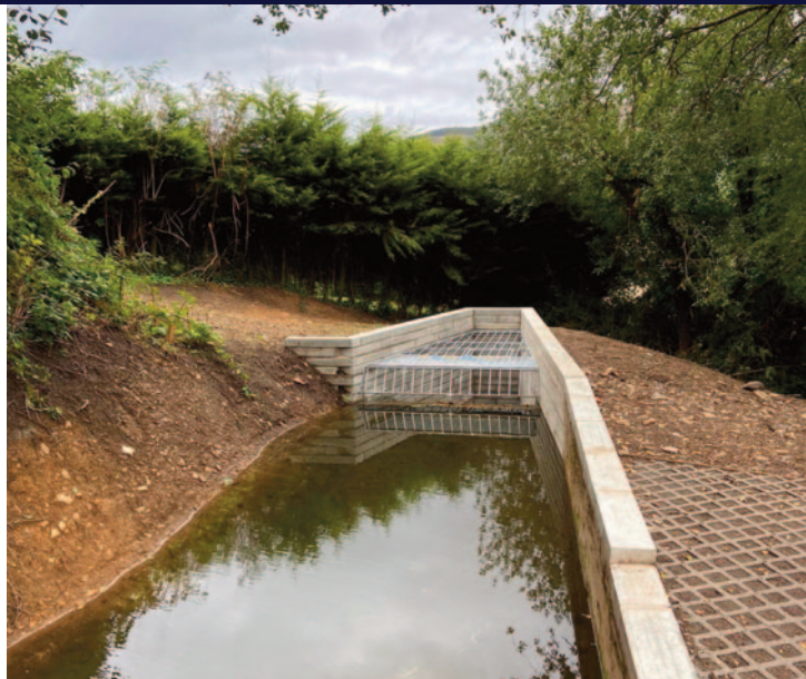
Culvert Inlet Improvement – Bryn Ifor, Mountain Ash
