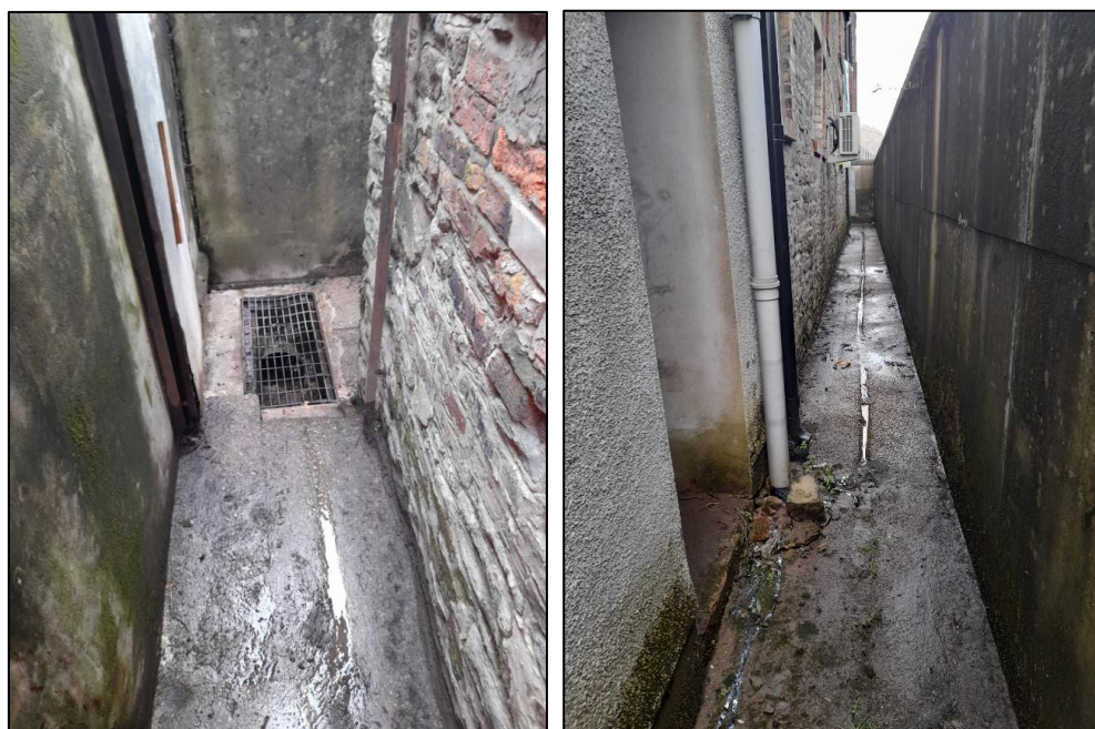
Figure 17: Image of the 'Surface Water Drain' (left) and the rear lane which discharges into the 'Surface Water Drain' behind commercial properties along Taff Street (right) (captured by an RCT FRM officer following Storm Bert).
