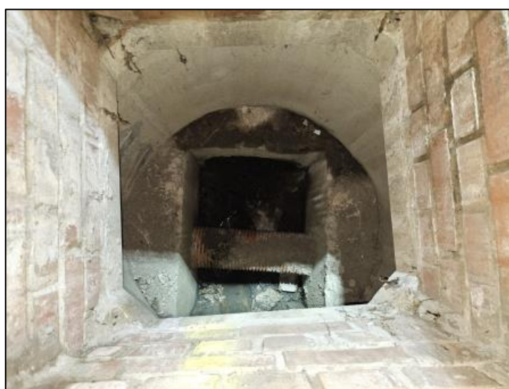
Figure 19: Image of the internal condition of 'Manhole 5' showing a DCWW combined sewer pipe crossing through the large diameter culvert (captured during CCTV operations in August 2025).
