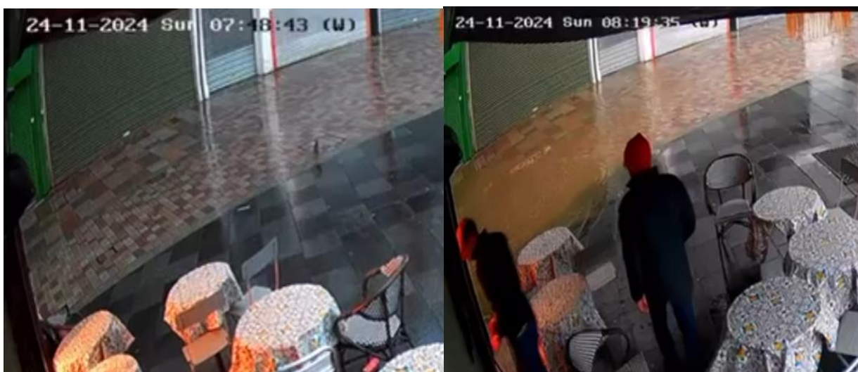
Figure 25: Image (left) showing Mill Street slot drain following the subsidence of heavy rainfall at 07:48 and image (right) at 08:19 showing surcharging over 30 minutes later.
