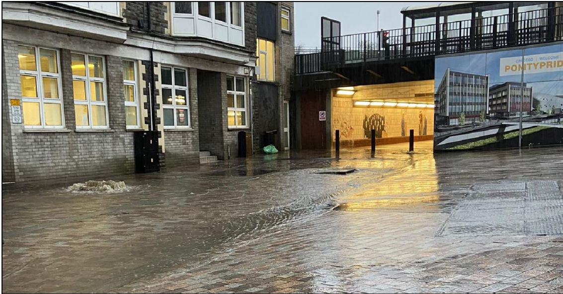
Figure 11: Image of ‘Manhole 2’ and ‘3’ associated to the combined sewer network at Mill Street surcharging during Storm Bert on Sunday 24 November 2024 (Image provided by business owner).
