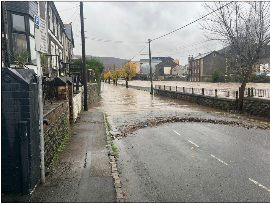
Figure 4: Image of the River Taf exceeding its channel capacity and overtopping the highway wall at Sion Street on the eastern river bank during the morning of Sunday 24 November 2024 (image captured by RCT FRM officer).
