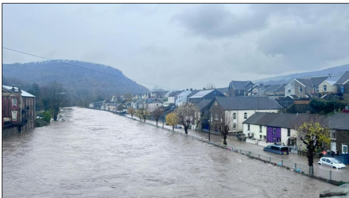
Figure 3: Image of the River Taf exceeding its channel capacity and overtopping the highway wall at Sion Street on the eastern river bank during Storm Bert (Image: BBC News).
