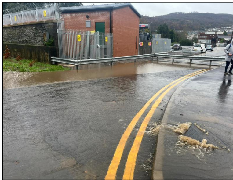
Figure 16: Image of 'Manhole 5' surcharging at Gas Road Car Park, Taff Street during Storm Bert (captured by an RCT FRM officer on 24 November 2024).
