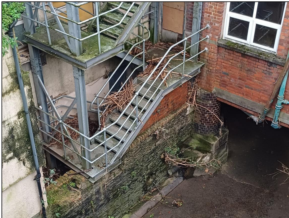
Figure 14: Image showing debris deposited by the River Rhondda on fire exit steps outside the basement and ground level of a commercial property at Mill Street (image captured by RCT FRM officer on 25 November 2024).
