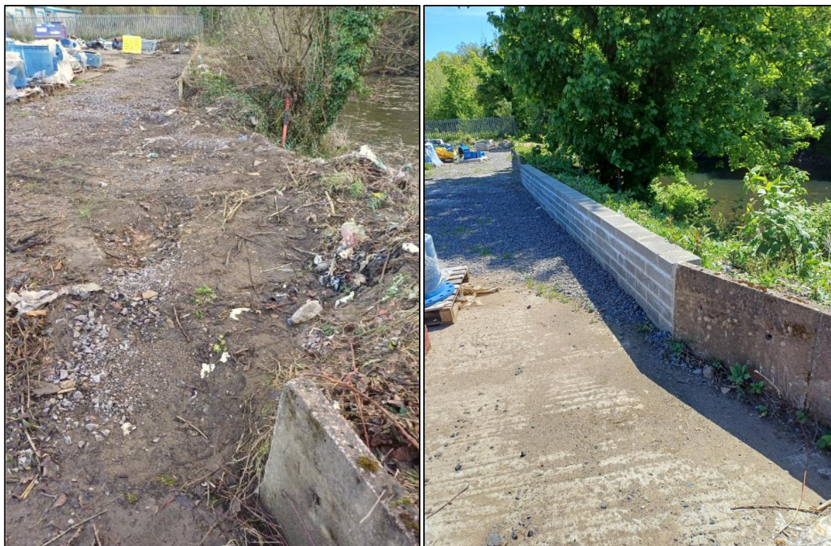
Figure 9: (Left) Gap created downstream of NRW flood defence wall by unpermitted removal of service crossing (image captured on 28/11/2024). (Right) New wall constructed to infill the gap downstream of NRW flood defence wall (image capture on 06/05/2025).
