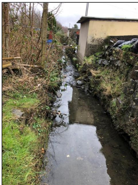
**Figure 22:** Evidence of stripped topsoil on the embankments of the unnamed ordinary watercourse to the rear of Gloucester Street (captured by RCT officers post storm event)
