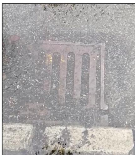
**Figure 31:** Blocked highway drainage gullies and ponding surface water along the unadopted road to the west of Abernant Road (captured by RCT officers post event)
