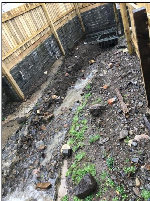
**Figure 10:** Evidence of deposited silt and debris within the unnamed ordinary watercourse channel and culvert inlet during post event inspection (captured by RCT's Flood Risk Management team on 21/02/2020)
