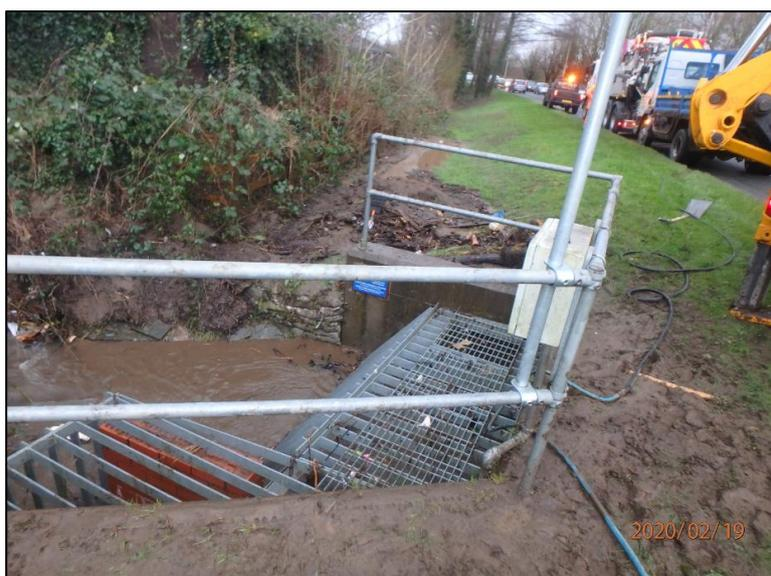
**Figure 11:** Image of 'Culvert Inlet 3' captured post event during cleansing operations (captured by RCT officers on 19<sup>th</sup> February 2020)
