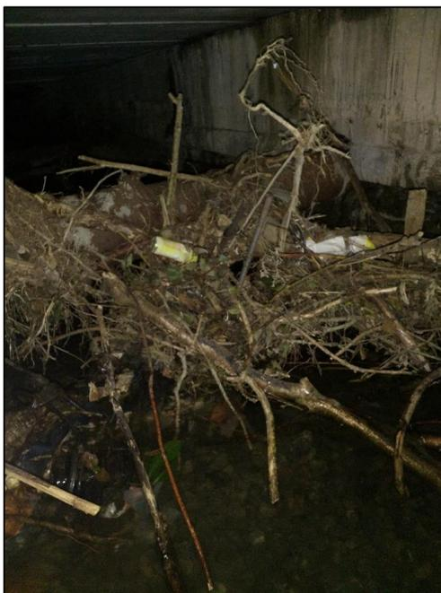
**Figure 17:** Large woody debris identified within the culvert network downstream of the culvert inlet adjacent to the B4275 (Cardiff Road) (captured during CCTV surveying operations)
