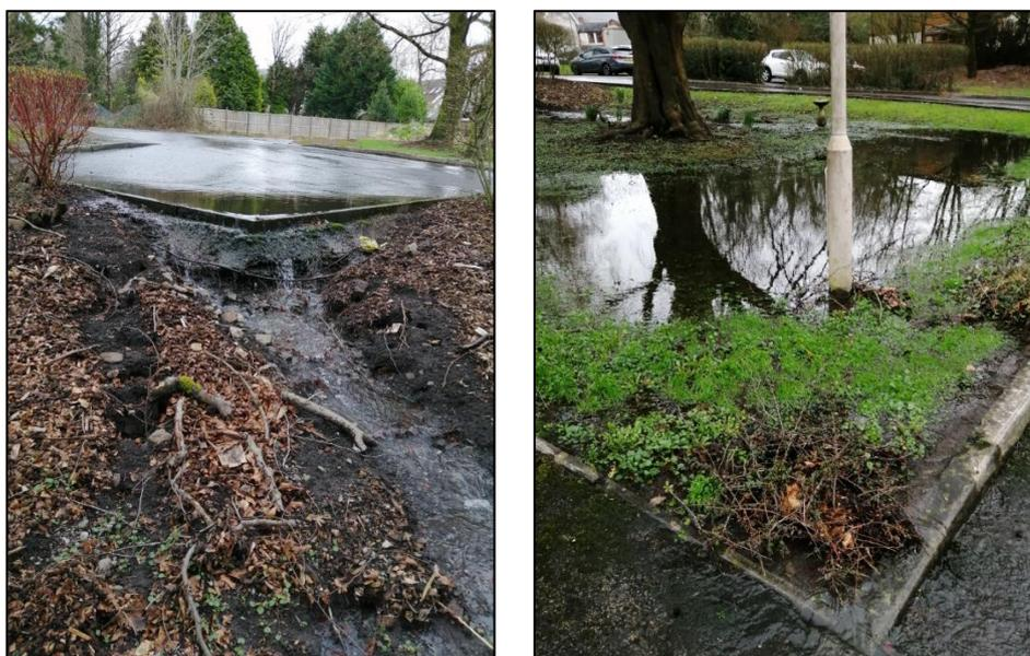
**Figure 4:** Evidence of surface water ponding and runoff within localised low points at Abernant Road (captured by RCT officers post Storm Dennis)
