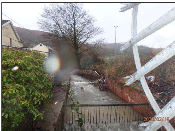
**Figure 27:** Deposition of material and scouring to the eastern embankment of the Nant Gwawr ordinary watercourse adjacent to Gwawr Street (captured by RCT officers on 18<sup>th</sup> February 2020)
