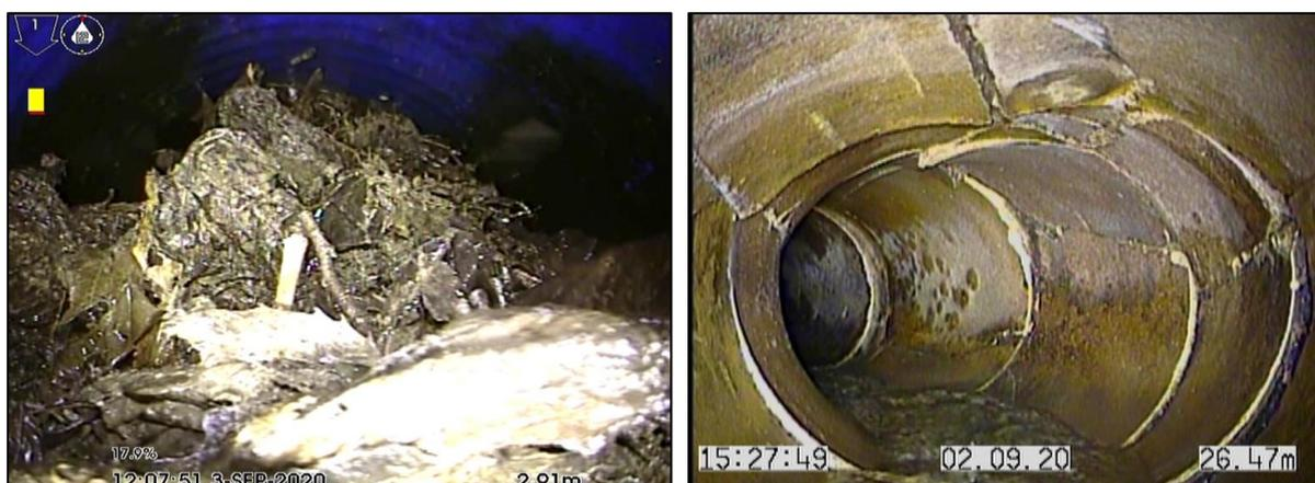
**Figure 15:** Debris accumulation upstream of 'Manhole 1' (left) and deformed overflow culvert network downstream of 'Manhole 1' (right) (captured during post event CCTV surveying operations)
