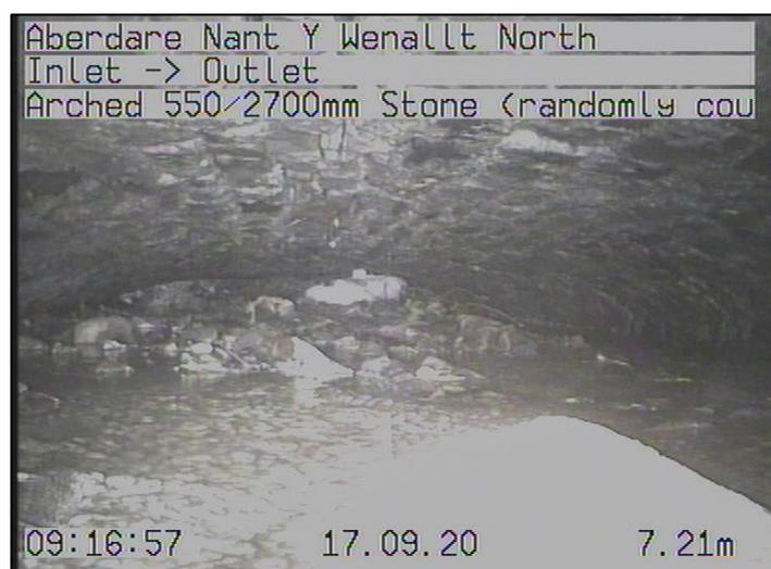
**Figure 14:** Evidence of settled debris within the 'Nant y Wenallt' culvert network downstream of 'Culvert Inlet 1' (captured during post event CCTV surveying)
