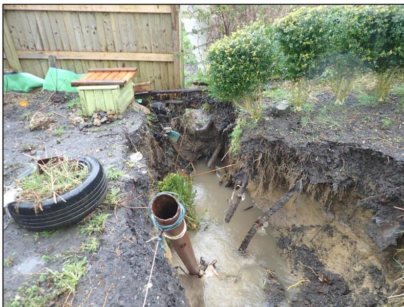
**Figure 5:** Collapsed culvert in the rear garden of Maeshyfyrd identified by RCT's Flood Risk Management team on 10/02/2020
