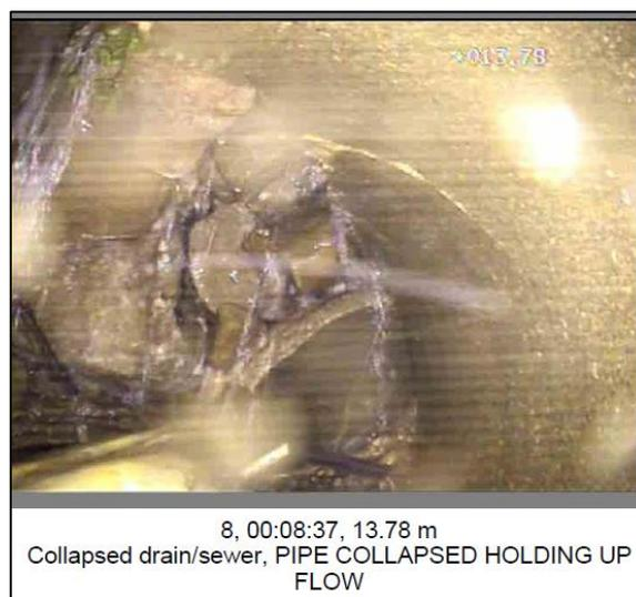
**Figure 17:** CCTV image of the collapsed 'Bryngolwg - Bro Deg' culvert network 13.78 metres upstream of MHS1 (CCTV survey undertaken 02/03/2020)
