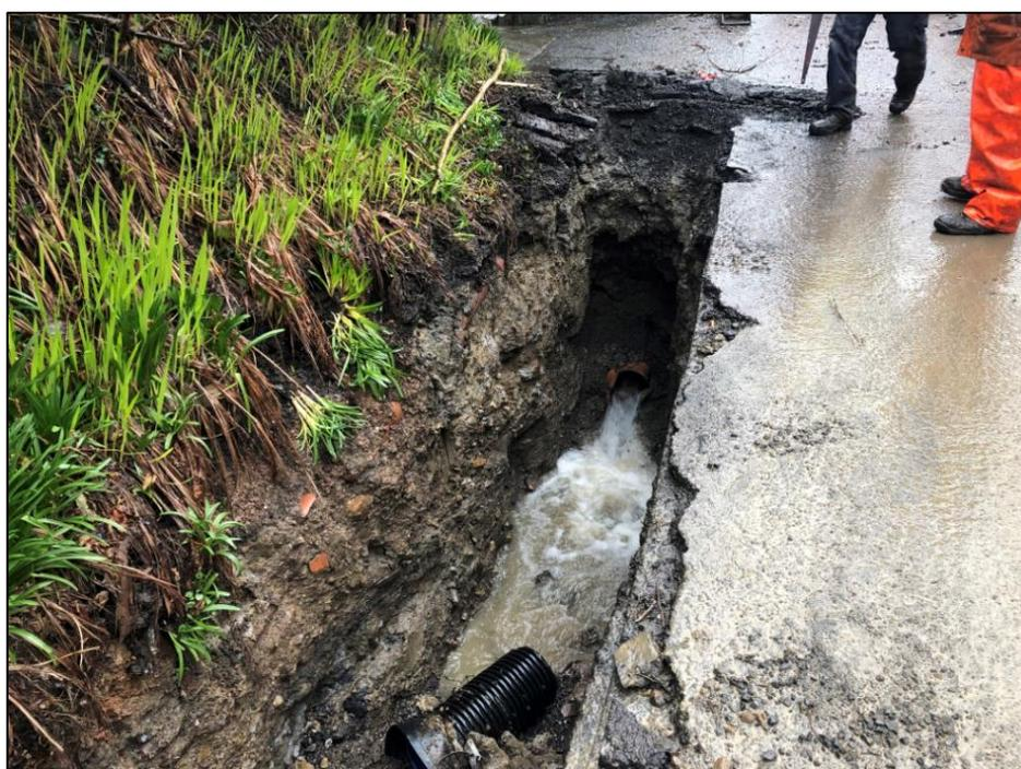
**Figure 11:** Collapsed culvert network ('Culvert Section 2') to the north of Cefnpennar Road identified during post event inspections (image captured by RCT's Flood Risk Management team on 18<sup>th</sup> February 2020)
