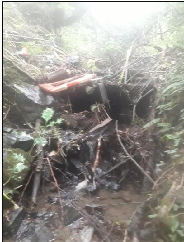
**Figure 28:** Woody debris and other material within the section of ordinary watercourse upstream of 'Culvert Inlet 1' at Tirfounder Road (captured during post event CCTV survey operations)
