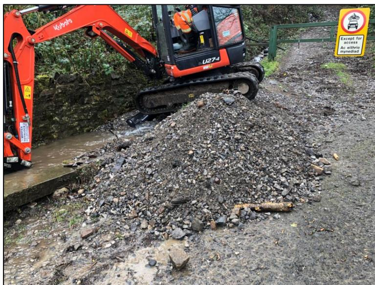
**Figure 23:** Silt and stone removed from the culvert inlets located upstream of the collapse at 'Culvert Section 2' along Cefnpennar Road (captured by RCT's FRM team on 18/02/2020)
