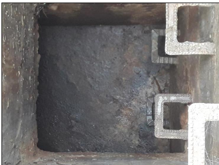
**Figure 25:** Significant volume of silt identified within 'Manhole 3' during CCTV survey operations (captured in June 2020)
