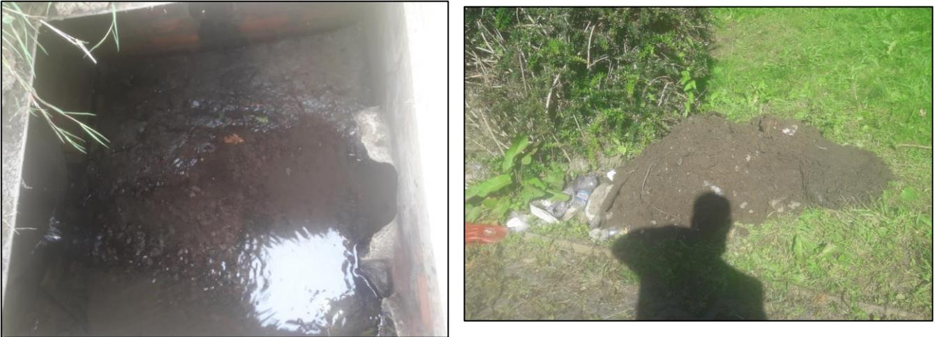
**Figure 19:** Mud and silt identified at MHS4 (Manhole 2, Figure 4) during CCTV survey operations prior to cleansing (left) and the debris removed from the MHS4 (right)
