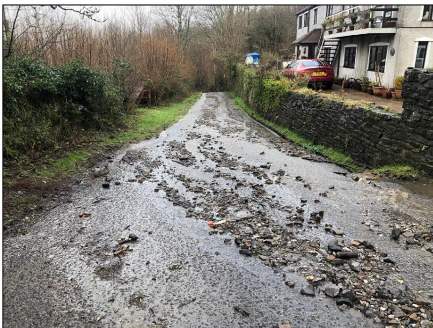
**Figure 35:** Debris deposited along Cefnpennar Road by surcharging watercourse and surface water flows during the storm event (image provided by resident)
