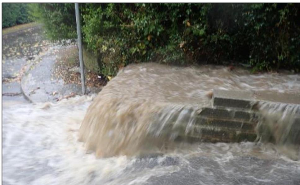
**Figure 12:** 'Culvert Inlet 2' at Cefnpennar Road surcharging and flooding onto the highway during Storm Dennis
