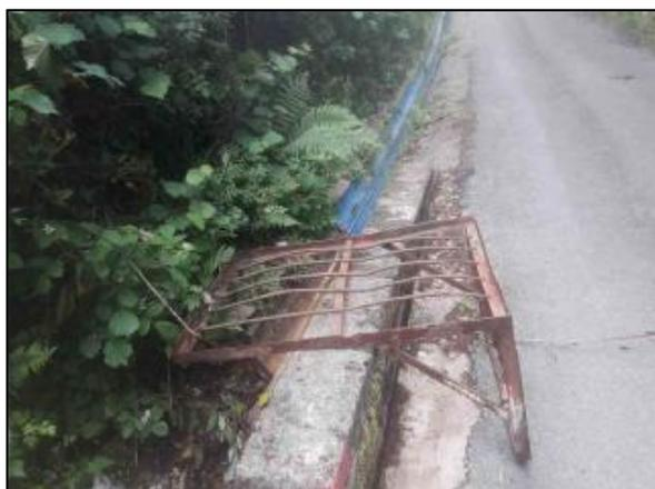
**Figure 21:** Damaged debris screen at 'Culvert Inlet 2' following Storm Dennis
