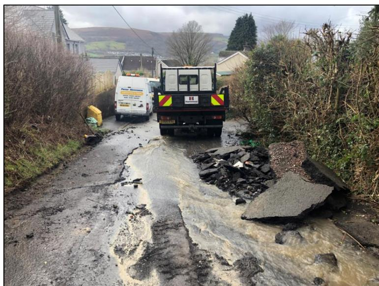
**Figure 24:** Downstream view of the culvert collapse which resulted in water flowing down Cefnpennar Road towards the lower reaches of Cwmbach (captured by RCT's FRM team on 18/02/2020)
