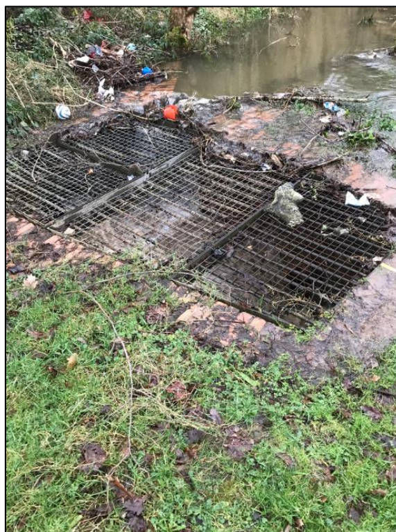
Figure 23: 'Culvert Inlet 8' blocked with debris and surcharging during Storm Dennis on 16 th February 2020 (image provided by resident)
