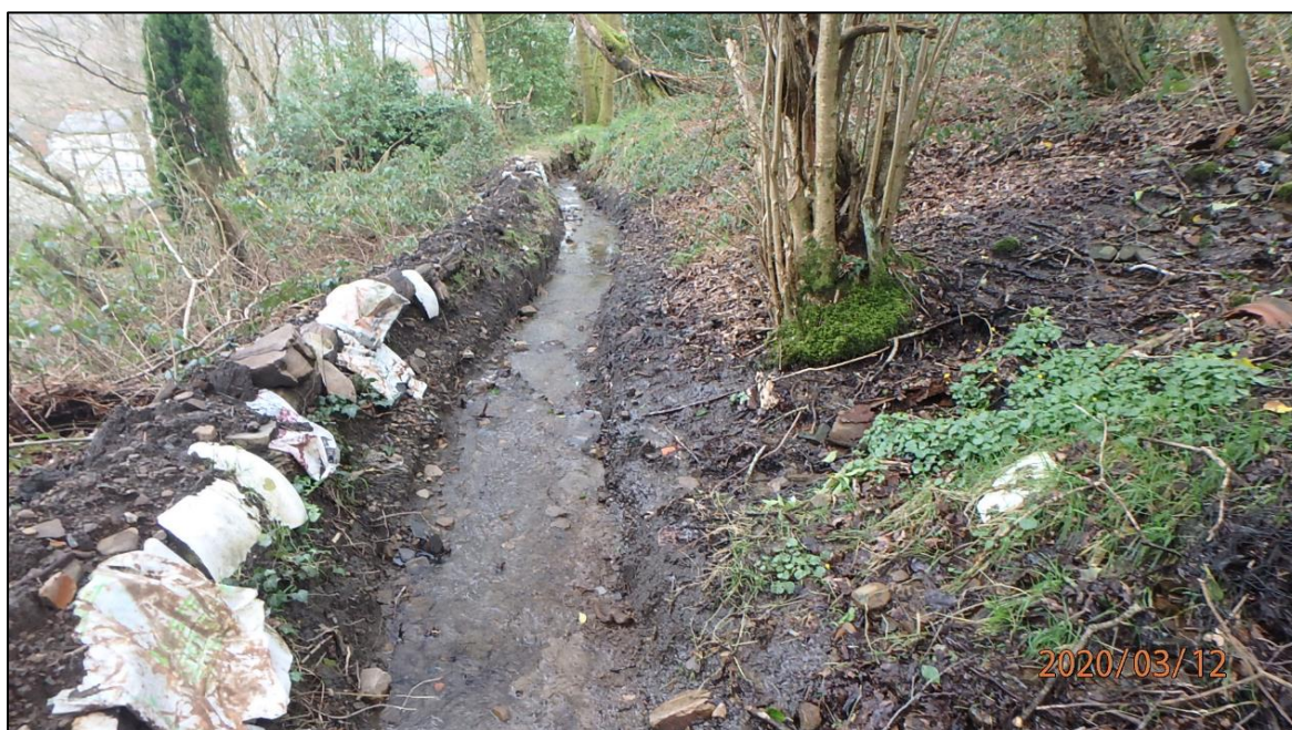
Figure 7: Open ditch that flows to the rear of Maple Terrace (captured by RCT's Flood Risk Management team on 12/03/20)
