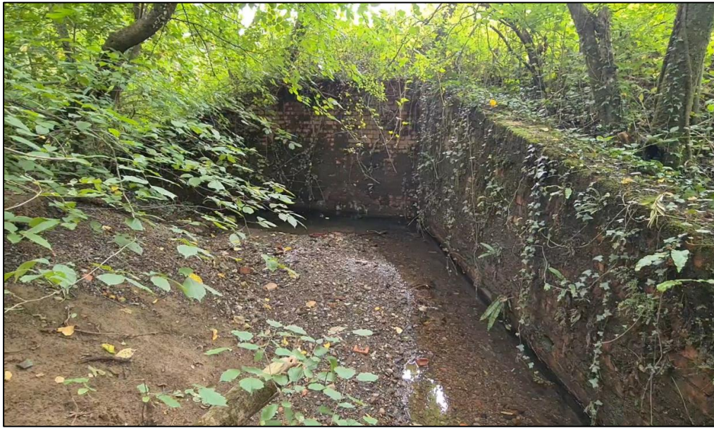
Figure 34: Photo of silt accumulation at the Glenboi culvert network outfall pond (captured by RCT during Storm Dennis on 16/02/2020)
