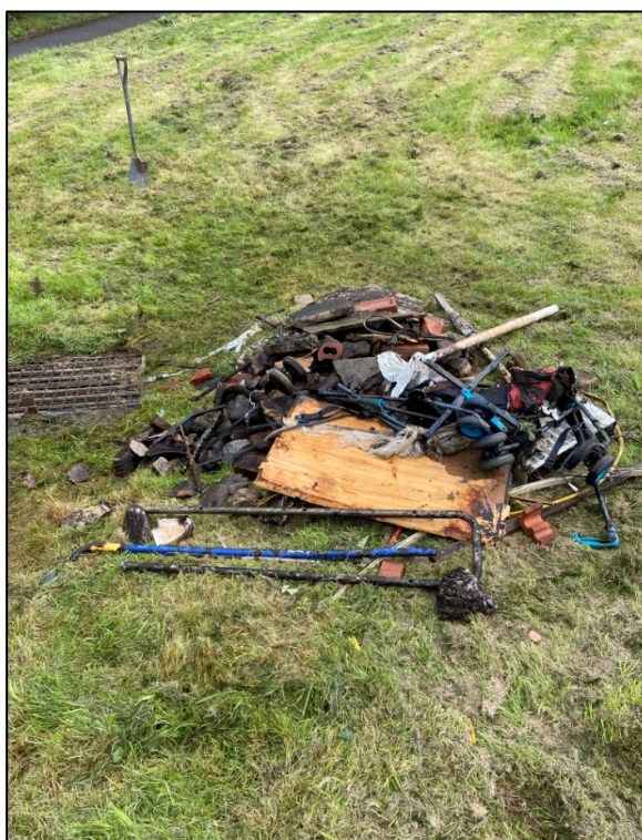
Figure 24: Debris removed from the ‘Glenboi’ culvert network following Storm Dennis during CCTV surveying and cleansing operations on 26/08/2020
