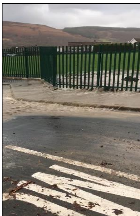
Figure 10: Image of 'Culvert Inlet 4' surcharging during Storm Dennis on 16 th February 2020 (image provided by resident)
