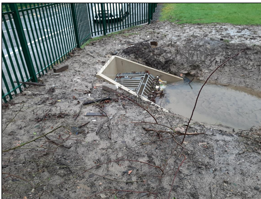
Figure 22: ‘Culvert Inlet 4’ captured after Storm Dennis by RCT’s Flood Risk Management team on 21st February 2020
