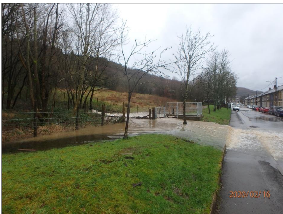
Figure 5: 'Culvert Inlet 1' surcharging at the inlet causing water to flow onto the highway and towards properties at Bronallt Terrace (captured by RCT's Flood Risk Management team on 16/02/2020)
