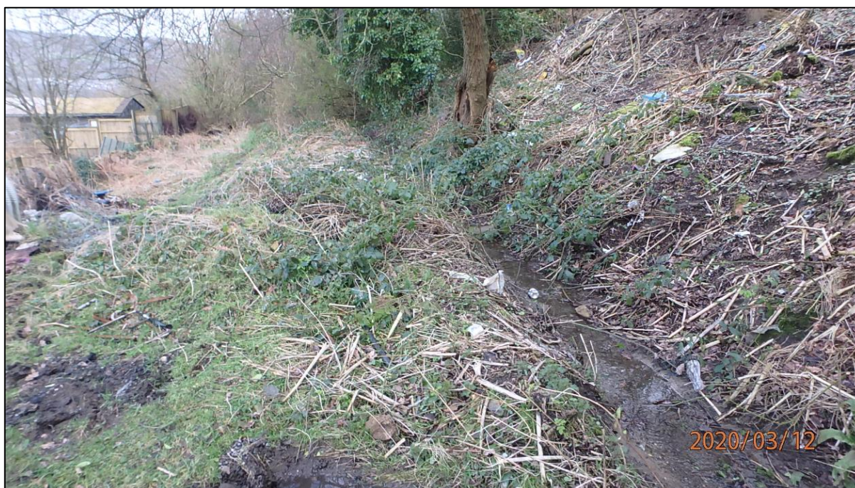
Figure 40: Evidence of flattened grass and mobilised debris indicative of overland flows down the hillside behind Maple Terrace during Storm Dennis (captured by RCT's Flood Risk Management team on 12/03/2020)
