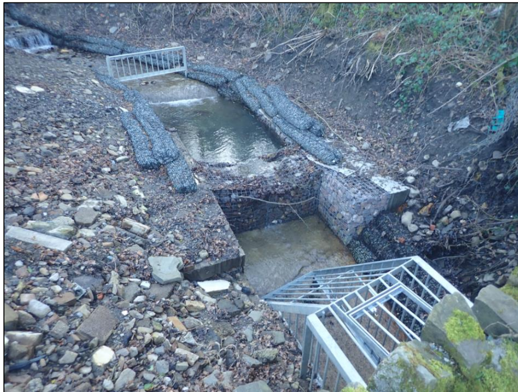
Figure 26: Open watercourse and upper catchment debris screens upstream of 'Pitt Cottages East Inlet' prior to Storm Dennis (captured by RCT's Flood Risk Management team on 06/02/2020)
