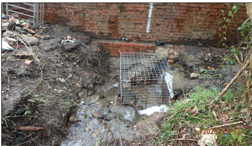
Figure 8: Mostyn Street culvert inlet (Culvert Inlet 2) following clearance works to remove the blockage (captured by RCT's Flood Risk Management team on 12/03/2020)
