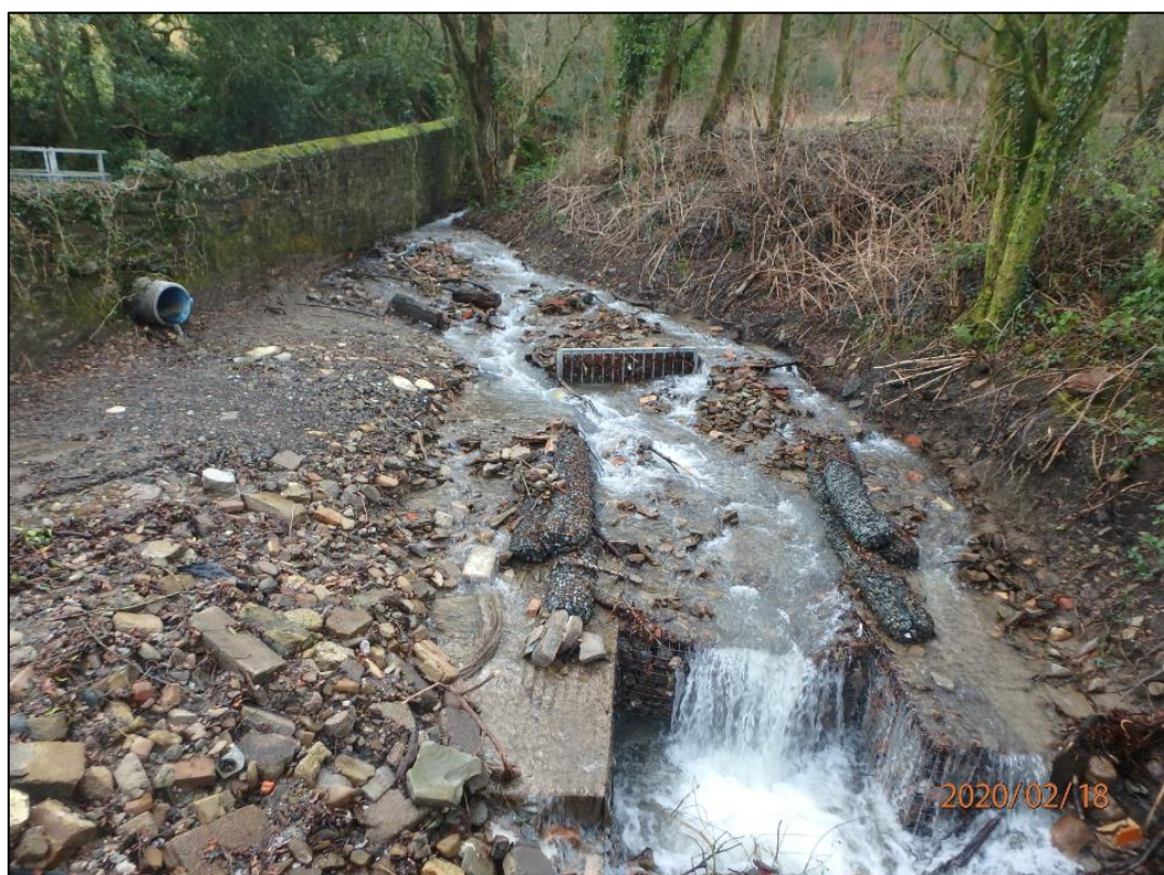
Figure 27: Open watercourse and upper catchment debris screens upstream of 'Pitt Cottages East Inlet' post Storm Dennis (captured by RCT's Flood Risk Management team on 18th February 2020)
