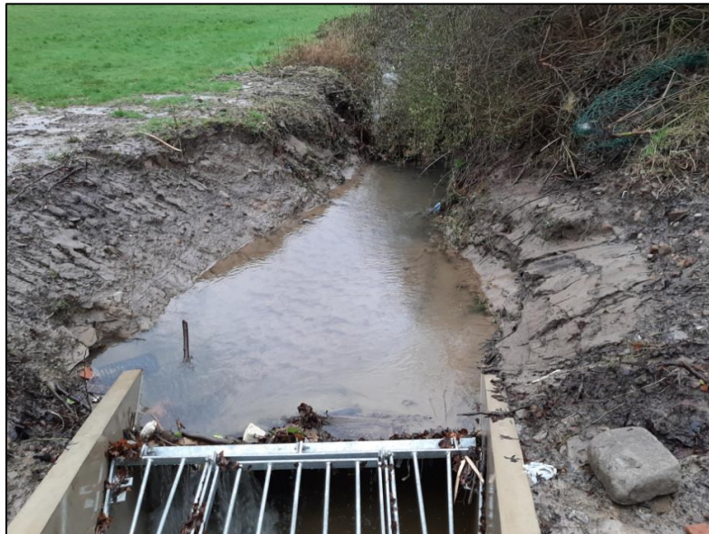
Figure 32: Condition of the open watercourse upstream of 'Culvert Inlet 4' captured post Storm Dennis (captured by RCT's Flood Risk Management team on 21/02/2020)
