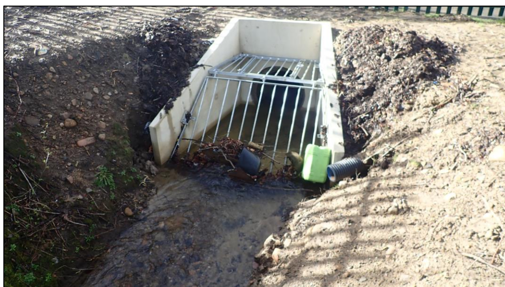
Figure 21: 'Culvert Inlet 4' captured before Storm Dennis by RCT's Flood Risk Management team on 13 th February 2020
