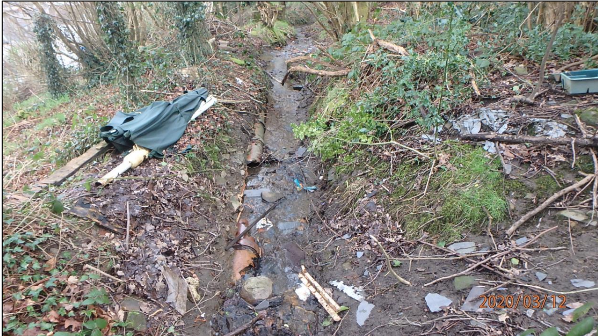
Figure 30: Cracked pipework within the open ditch and various pieces of debris within the channel and surrounding area (captured by RCT's Flood Risk Management team on 12/03/20)
