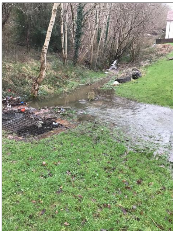
Figure 12: 'Culvert Inlet 8' surcharging during Storm Dennis on 16 th February 2020 (image provided by resident)
