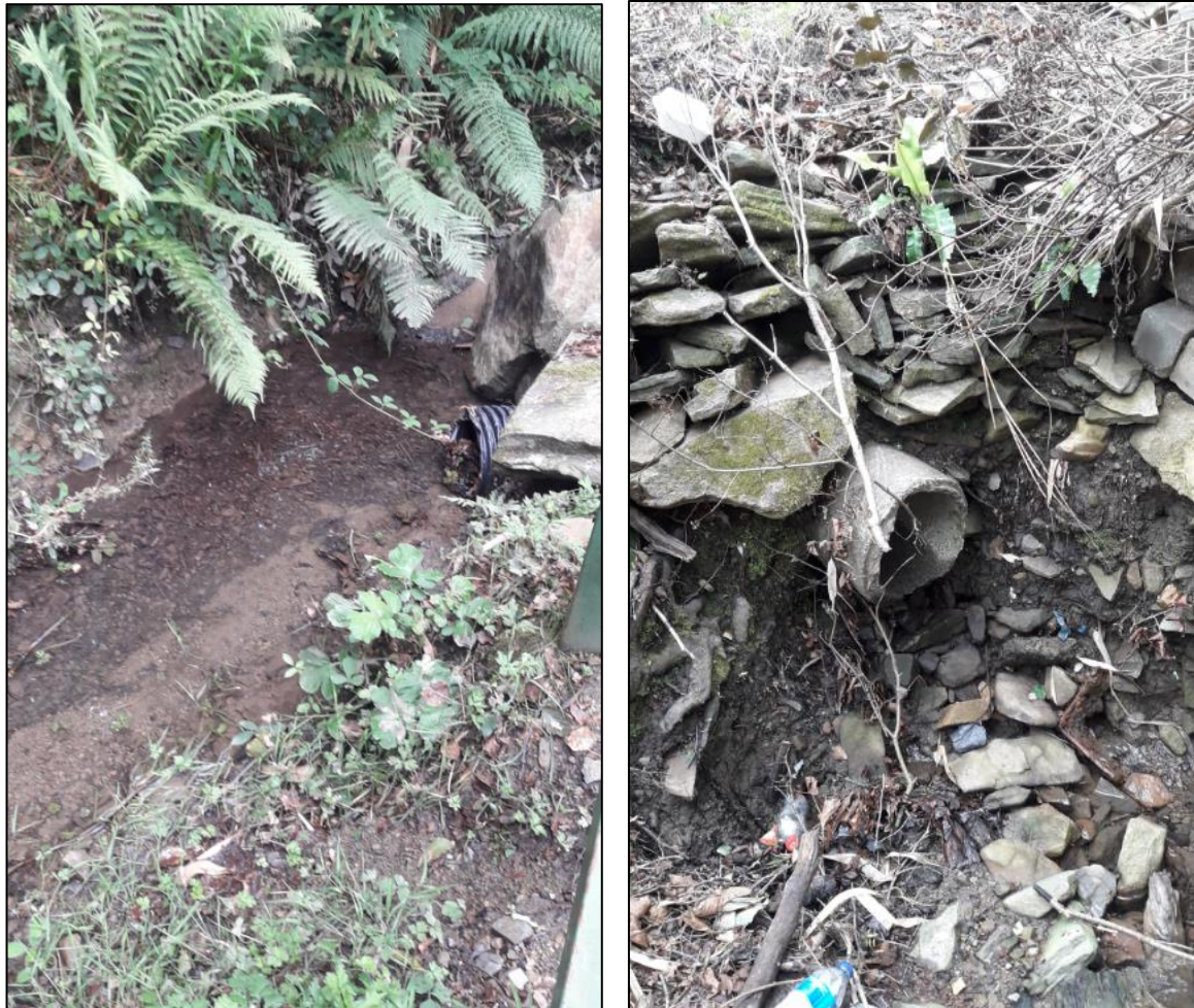
Figure 20: 'Culvert Inlet 3' (left) and outlet (right) at Sierra Pines captured post storm event (images provided by NRW)
