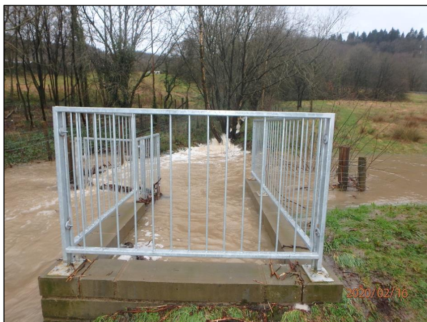
Figure 16: 'Culvert Inlet 1' surcharging during Storm Dennis on 16 th February 2020 (captured by RCT's Flood Risk Management team)
