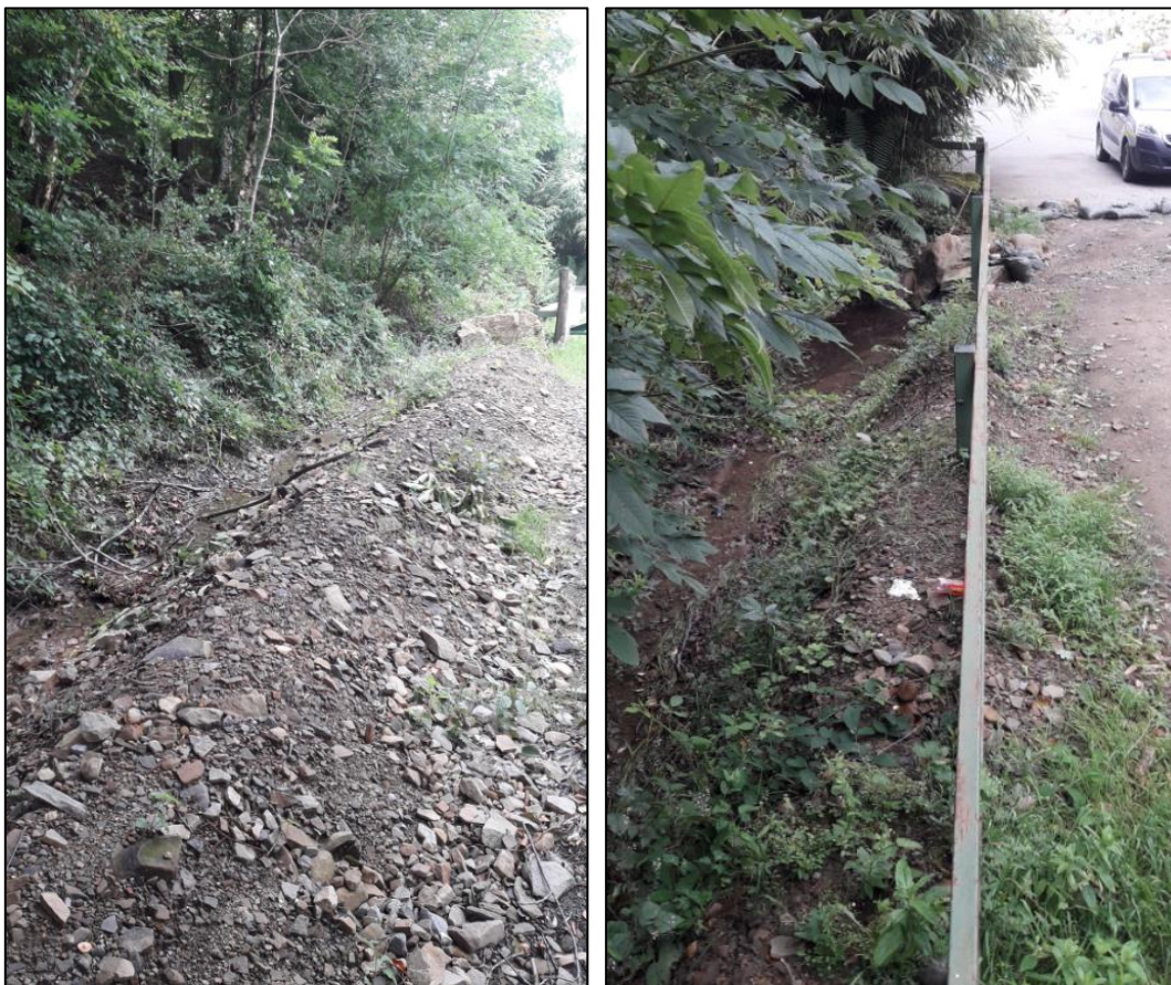
Figure 31: Land drainage channel adjacent to the St Gwynno forestry access road which feeds into ‘Culvert Inlet 3’
