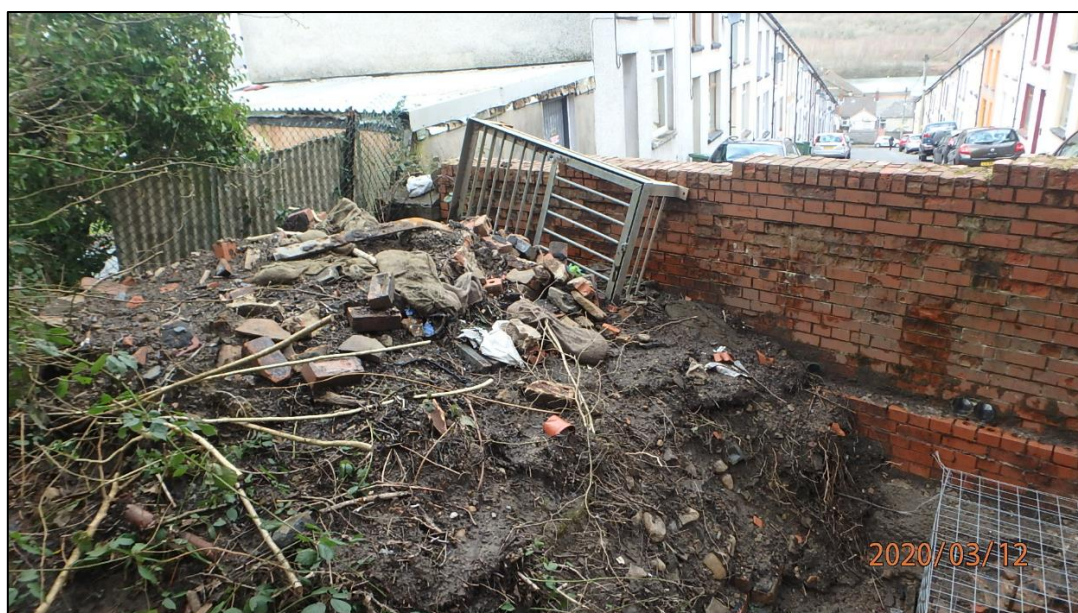
Figure 18: Debris and former inlet debris screen removed from 'Culvert Inlet 2' by RCT's Highways and Streetcare Depot following Storm Dennis (image captured by RCT's FRM officer on 12/03/2020)
