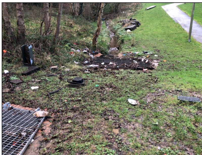
Figure 33: Open watercourse upstream of 'Culvert Inlet 8' captured post Storm Dennis (captured by RCT's Flood Risk Management team on 25/02/2020)
