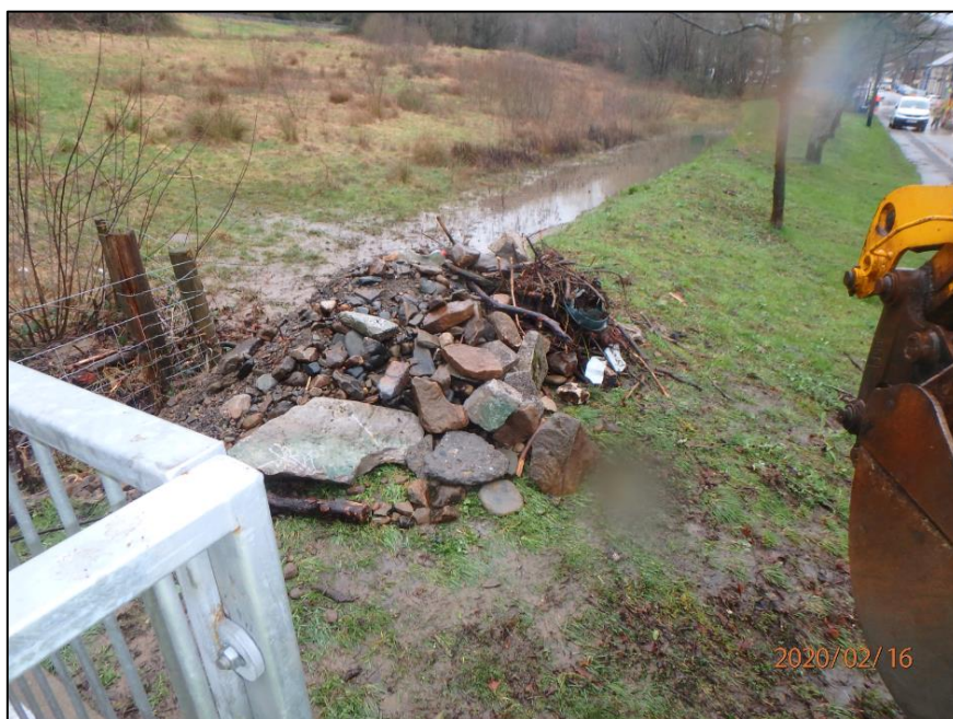
Figure 17: Debris removed from 'Culvert Inlet 1' which was identified as surcharging during Storm Dennis on 16 th February 2020 (captured by RCT's Flood Risk Management team)
