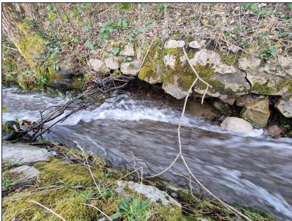
Figure 28: Image depicting a small area of scour within the unnamed open watercourse upstream of 'Culvert Inlet 1' (captured by RCT's Flood Risk Management team post Storm Dennis)
