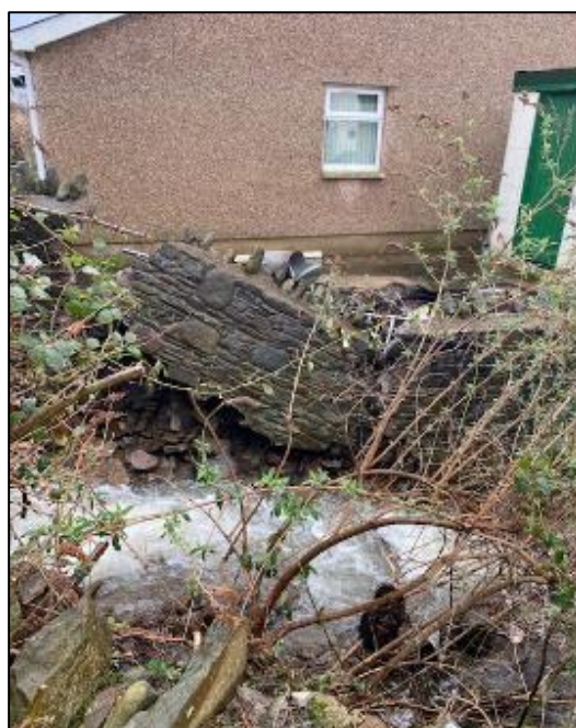
Figure 30: Evidence of damaged channel retaining wall within Area 2, Figure 26, of the Nant y Ffrwd ordinary watercourse (captured by RCT's Flood Risk Management team during post storm investigations)
