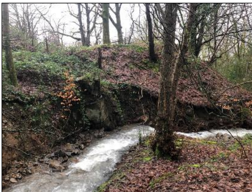
Figure 27: Photo of significant embankment scour and undercutting to the Nant y Ffrwd ordinary watercourse within Area 1, Figure 26 (captured by RCT's Flood Risk Management team on 25/02/2020)
