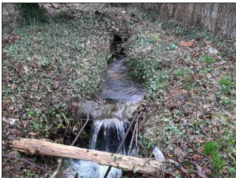
Figure 32: 'Unnamed ordinary watercourse 1' upstream of 'Culvert Inlet 2' captured by RCT officers post event
