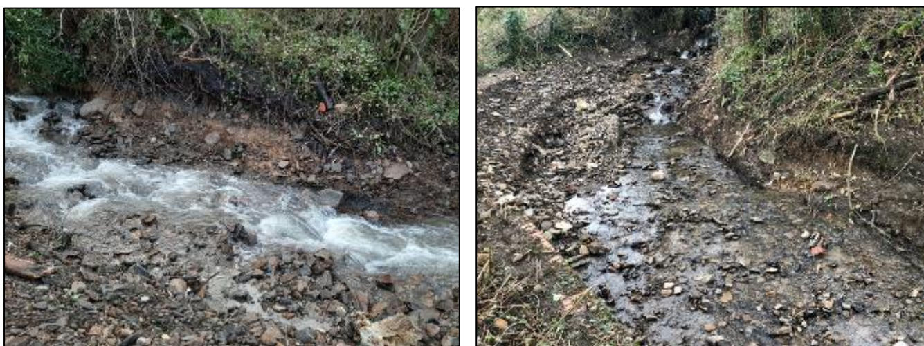
Figure 34: Evidence of embankment erosion (left) and deposition of material (right) within ‘unnamed ordinary watercourse 3’ upstream of ‘Culvert Inlet 6’ (captured by RCT officers on 29 th February 2020)
