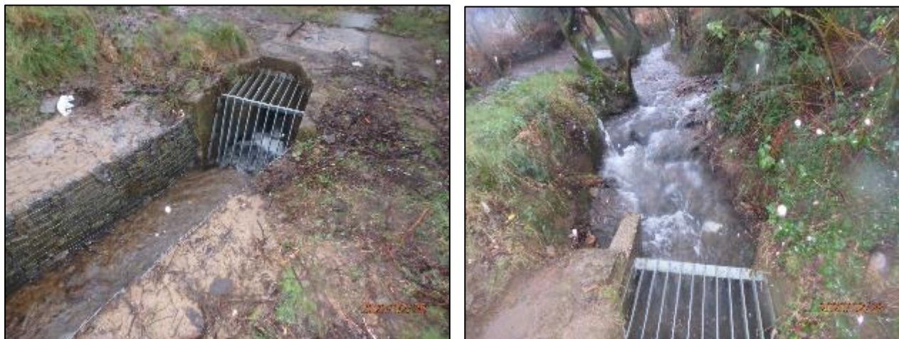
Figure 22: ‘Culvert Inlet 3’ (left) and ‘Culvert Inlet 5’ (right) structures captured post Storm Dennis
