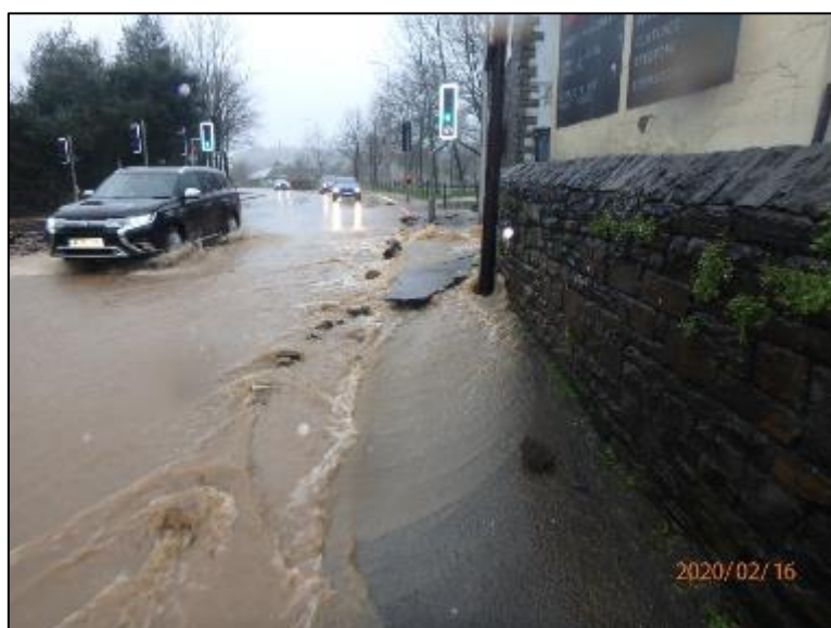
Figure 7: Evidence of flood water discharging from a damaged section of footpath adjacent to the A4059 (New Road) and conveying onto the highway during Storm Dennis (captured by RCT officers on 16 th February 2020)
