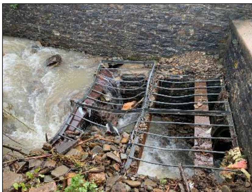
Figure 6: Evidence of damage to ‘Culvert Inlet 1’ at Campbell Terrace identified during post storm investigations (captured by RCT’s Flood Risk Management team on 18 th February 2020)
