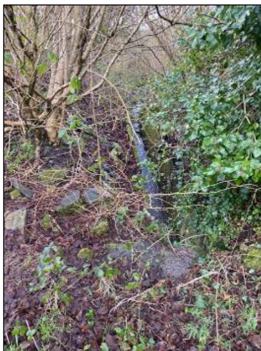
Figure 9: Evidence of an ordinary watercourse present along the hillside to the rear of Clas-y-Dderwen. (Captured by RCT's Flood Risk Management team during post storm investigations)
