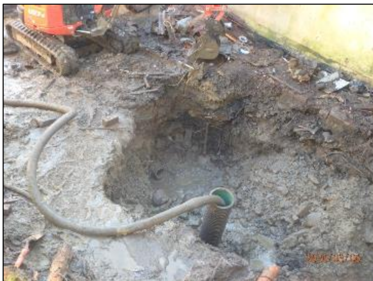
Figure 23: Collapsed culvert pipework downstream of 'Culvert Inlet 4' which was identified as buried during emergency repair works (captured by RCT officers post Storm Dennis)
