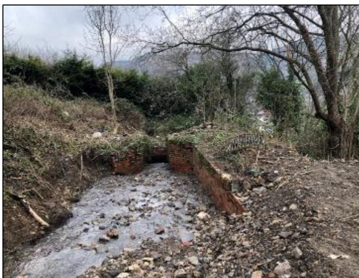
Figure 24: Evidence of flattened grass and deposits of debris at 'Culvert Inlet 6' post event (captured by RCT officers)
