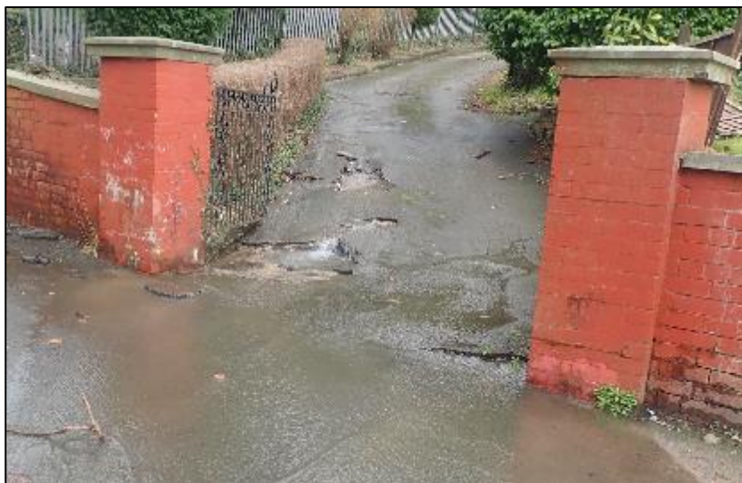
Figure 8: Evidence of surface water scour on the driveway of a residential property at Aber-ffrwd Road (Captured by RCT’s Flood Risk Management team during post storm investigations)
