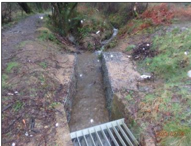
Figure 33: 'Unnamed ordinary watercourse 2' upstream of 'Culvert Inlet 3' captured by RCT officers post event
