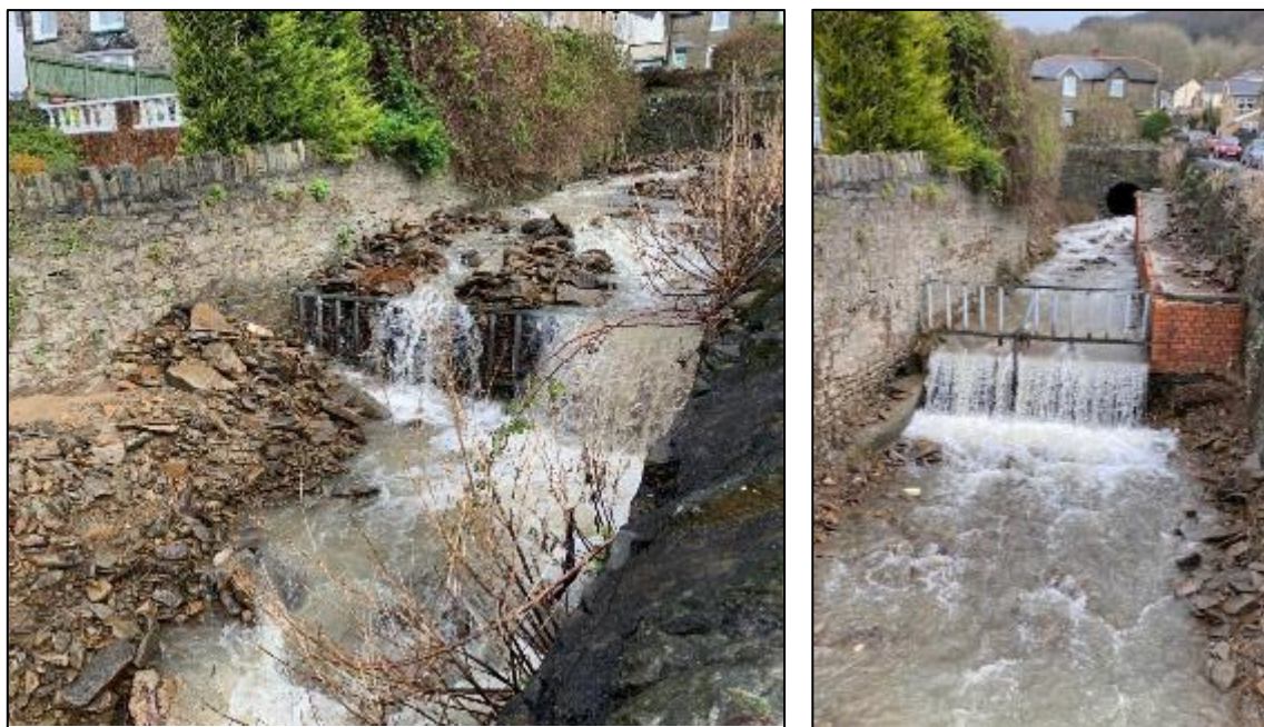
Figure 29: A comparison of the Nant y Ffrwd open watercourse channel, adjacent to Allen Street within Area 2, Figure 26, pre (left) and post (right) clearance of debris material (captured by RCT’s Flood Risk Management team on 18/02/2020 (left) and 01/03/2020 (right))
