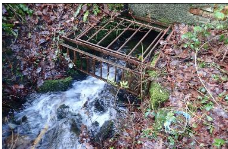
Figure 20: 'Culvert Inlet 2' captured prior to Storm Dennis (captured by RCT's Flood Risk Management team on 13 th February 2020)
