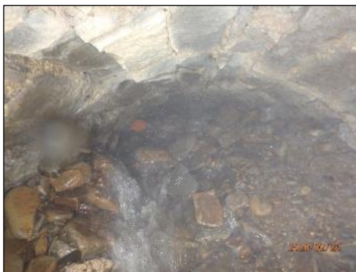
Figure 19: Settled debris deposits identified within the 'Nant y Ffrwd Culvert Network' downstream of 'Manhole 1' during CCTV survey, jetting and cleansing operations on 26 th February 2020
