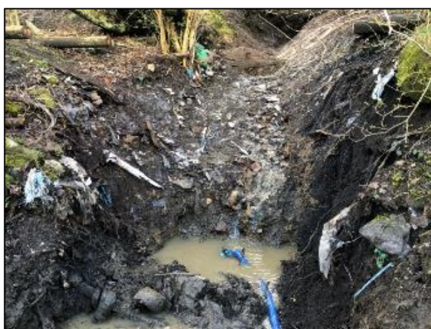
Figure 13: Ordinary watercourse channel upstream of 'Culvert Inlet 4' and evidence of ponding water on top of buried 'Culvert Inlet 4' during post event inspections (captured by RCT's Flood Risk Management team)
