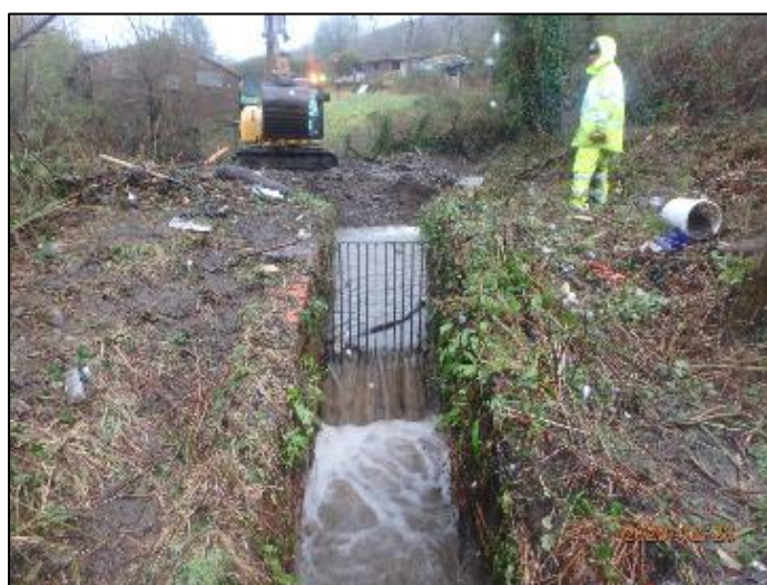
Figure 14: 'Culvert Inlet 6' at Bryn lfor during emergency clearance works following Storm Dennis (captured by RCT's Flood Risk Management team on 28 th February 2020)
