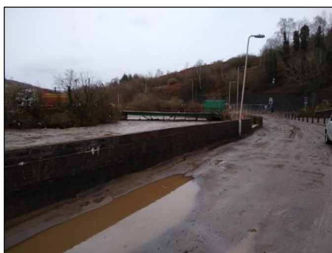
Figure 6: Evidence of riverine mud and silt at Brook Street following the overtopping of the River Rhondda during Storm Dennis (image provided by resident and captured on 16 th February 2020)
