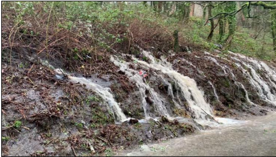
Figure 9: Overland flow travelling down the hillside from Leslie Terrace and conveying towards the rear of Llwynceilyn Industrial Estate during the storm event (image provided by business owner)
