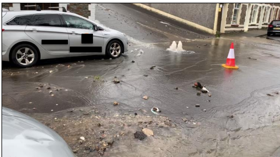
Figure 12: Evidence of 'Manhole 1' surcharging at Leslie Terrace during Storm Dennis (image provided by business owner)
