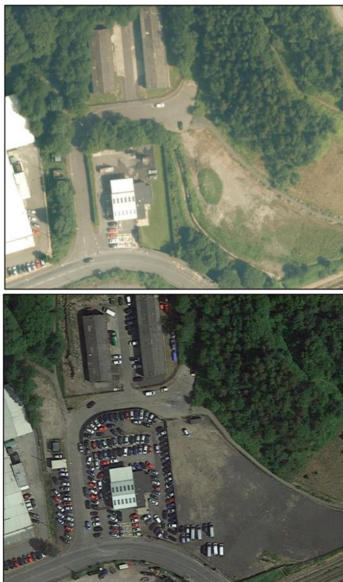
Figure 19: Aerial view of Llwynceilyn Industrial Estate in 2014 (top) and in 2020 (bottom)
