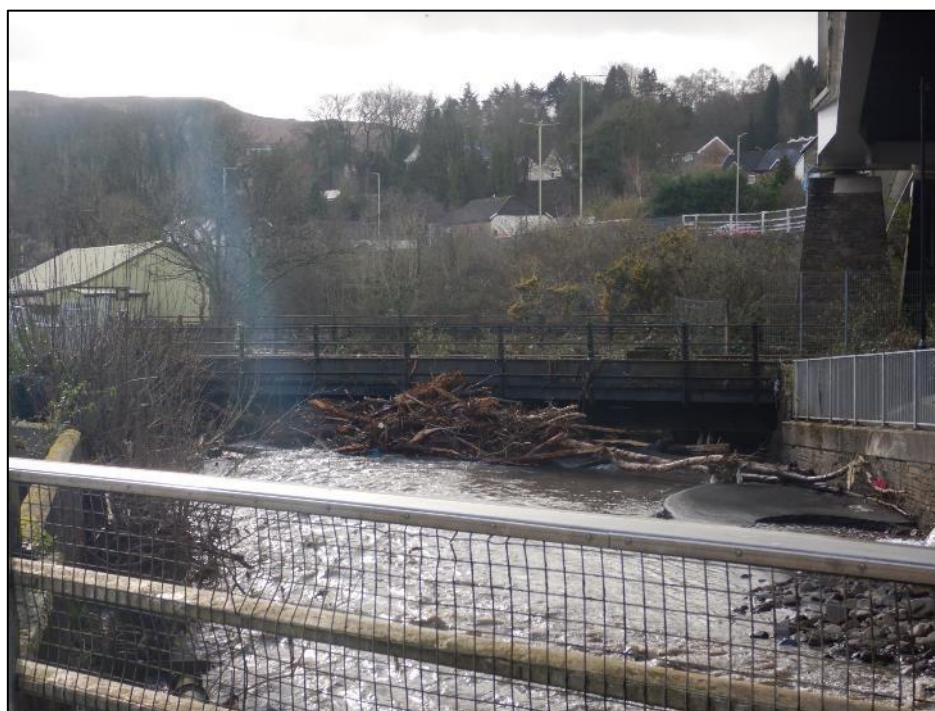
Figure 3: Image of obstruction at Rhondda Fach railway bridge (captured by RCT's Flood Risk Management team on 17 th February 2020)
