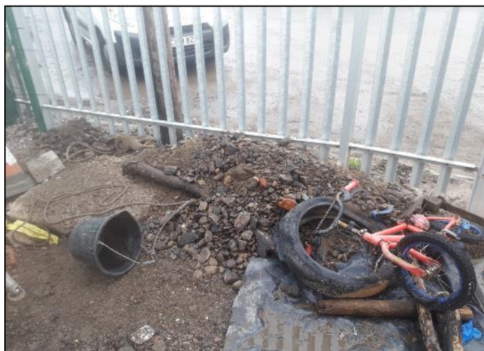
Figure 17: Material removed from the Nant Llwynceilyn culvert network downstream of 'Culvert Inlet 2' during cleansing operations
