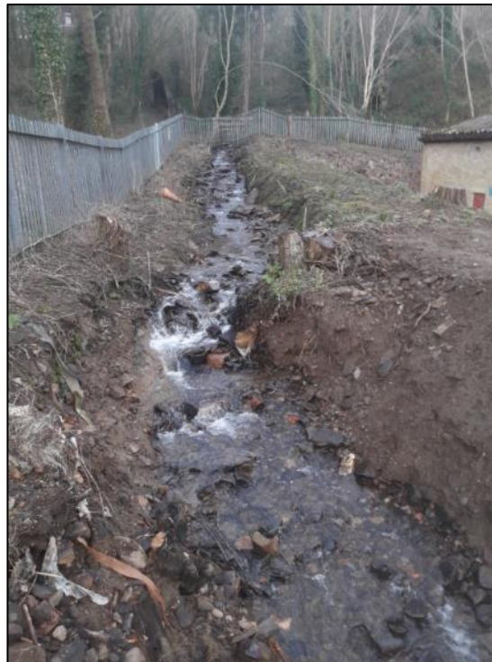
Figure 22: Nant Llwynceilyn ordinary watercourse upstream of 'Culvert Inlet 2' within Llwynceilyn Industrial Estate (captured during CCTV survey operations post Storm Dennis)
