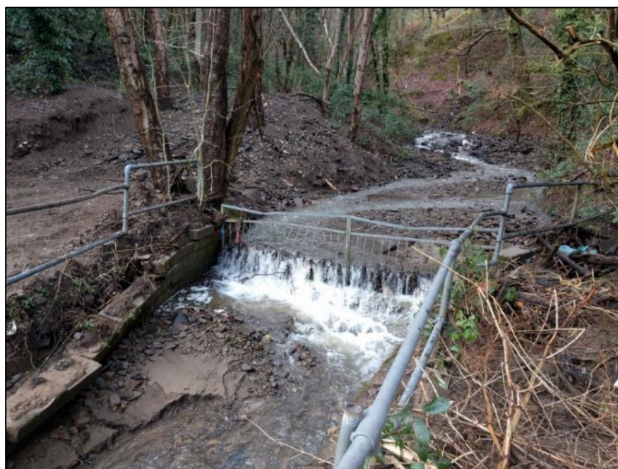
Figure 21: Upstream view of the Nant Llwynceilyn ordinary watercourse channel (captured by RCT's Flood Risk management team post Storm Dennis)
