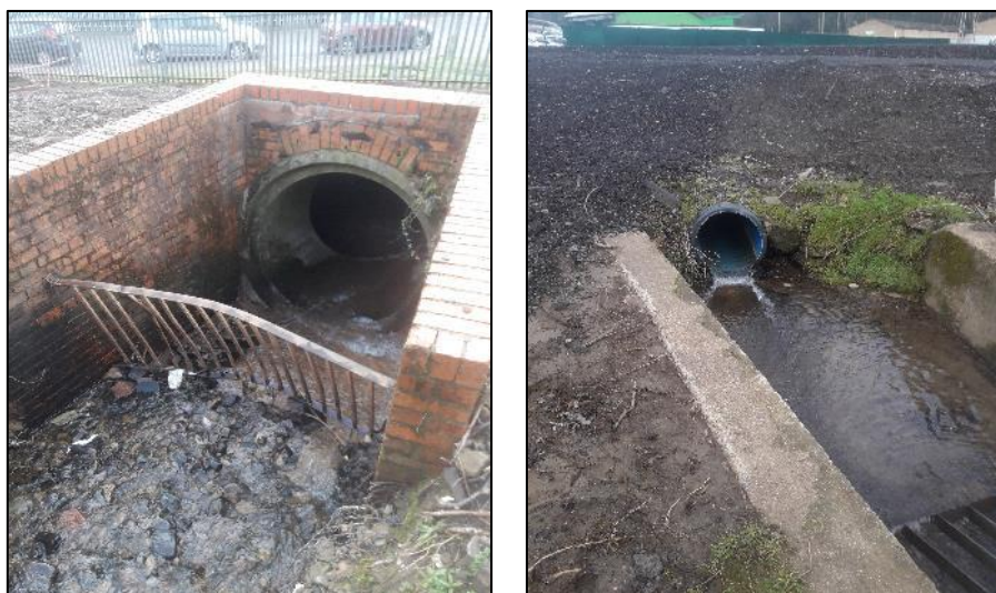
Figure 18: 'Culvert Inlet 2' consisting of a large 1.5 metre diameter concrete pipe (left) and the downstream outlet consisting of a 600mm diameter plastic pipe (captured by external surveying team post event)
