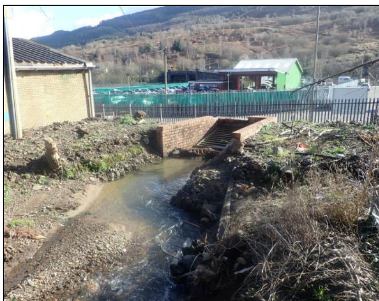
Figure 13: Post event condition of 'Culvert Inlet 2' which was identified as a source of flooding during Storm Dennis (image provided by business owner)
