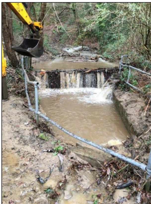
Figure 8: Post event condition of 'Culvert Inlet 1' which surcharged during Storm Dennis (image captured by RCT's Highway and Streetcare Depot on 16 th February 2020)
