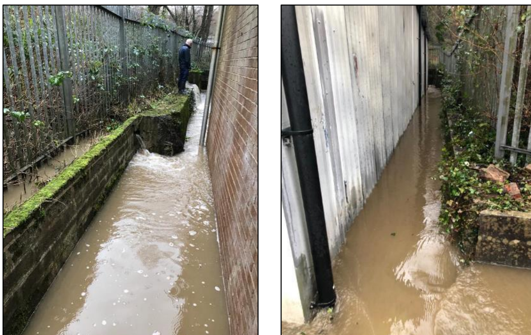
Figure 11: Ordinary watercourse and surface water flows causing external flooding to the rear of commercial units at Llwynycelyn Industrial Estate during Storm Dennis (image provided by business owner)
