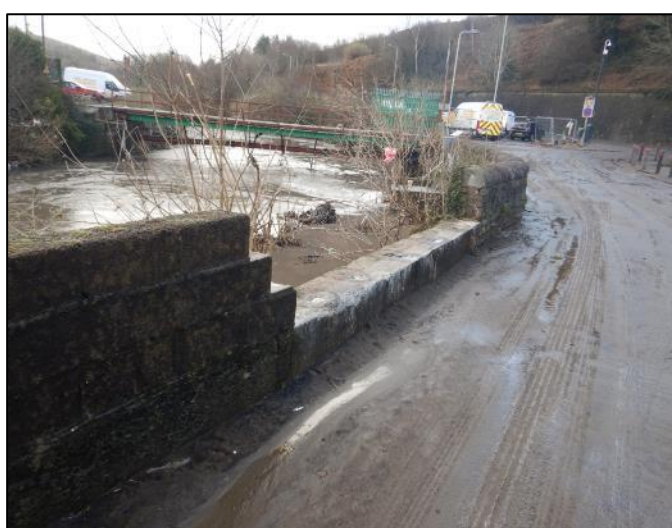
Figure 5: 8-metre-long section of collapsed retaining wall (NFD Structure) adjacent to the River Rhondda at Brook Street (image captured by RCT officers on 17 th February 2020)
