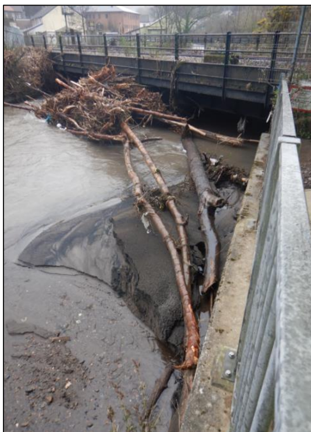
Figure 27: Accumulated debris within the Rhondda Fach River channel and at Rheola Bridge structure which caused a damming effect to the flow during Storm Dennis (captured by RCT officer on 17 th February 2020)
