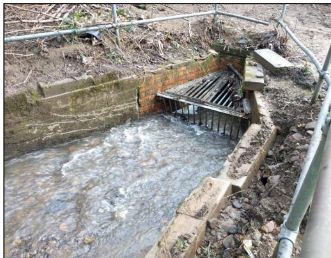
Figure 16: Image of 'Culvert Inlet 1' captured by RCT's Flood Risk Management team post event
