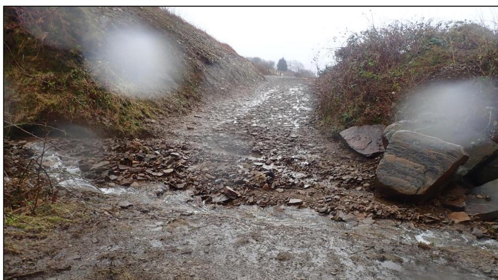
**Figure 14:** Overland flow and deposition of material across the hillside track above RCT20 (captured by RCT's Flood Risk Management team on 19/02/2020)
