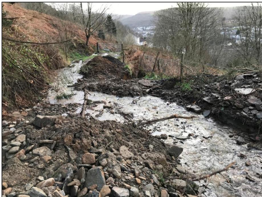
**Figure 16:** Significant deposition of scoured material along the hillside track above 'Culvert Inlet 2' post Storm Dennis (image provided by resident)
