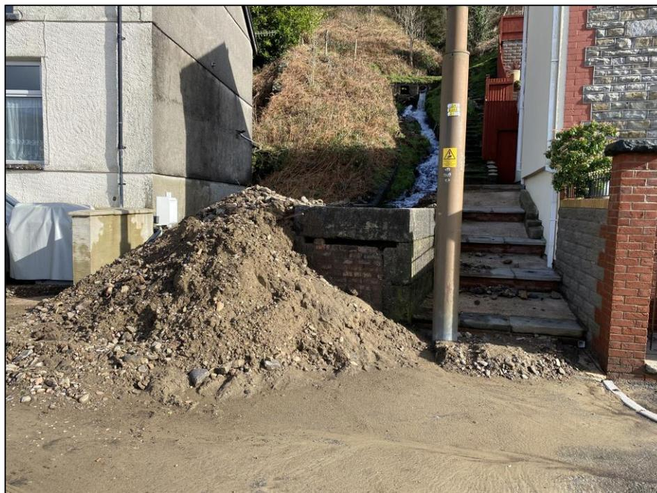
**Figure 7:** Post storm event photograph of 'Culvert Inlet 1' depicting the displacement of material (Image captured by a RCT's Flood Risk Management team on 17<sup>th</sup> February 2020)
