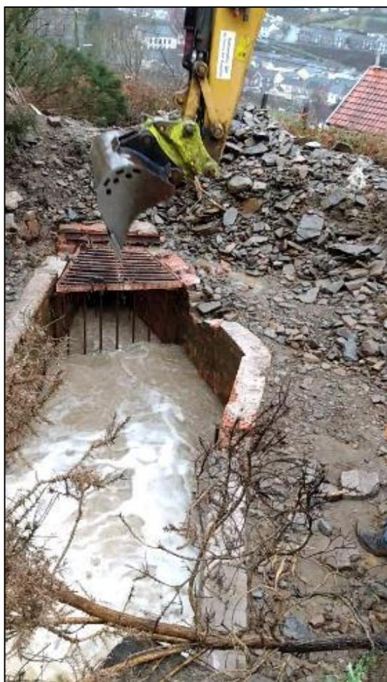
**Figure 11:** 'Culvert Inlet 2' being cleared of debris following Storm Dennis (image provided by resident and captured 16<sup>th</sup> February 2020)
