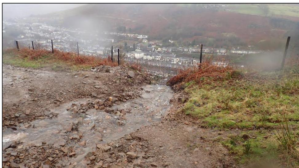
**Figure 13:** Overland flow travelling across the hillside track towards the hillside upstream of 'Culvert Inlet 1' (captured by RCT's Flood Risk Management team on 19/02/2020)
