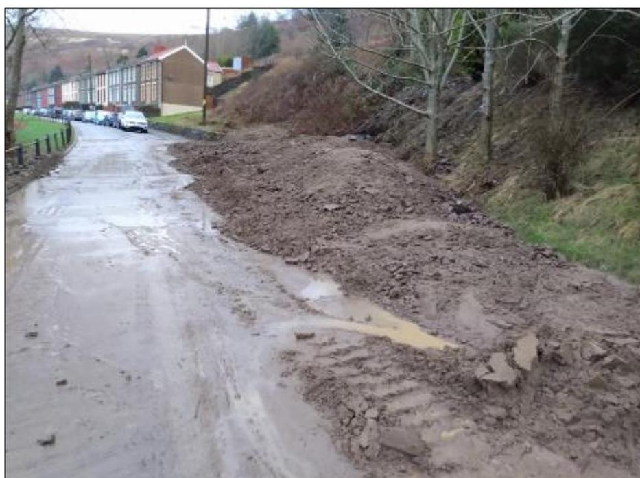
**Figure 22:** Mud, silt and debris deposited onto the highway at Heath Terrace following the clearance operation of 'Culvert Inlet 2' during Storm Dennis (image provided by resident)
