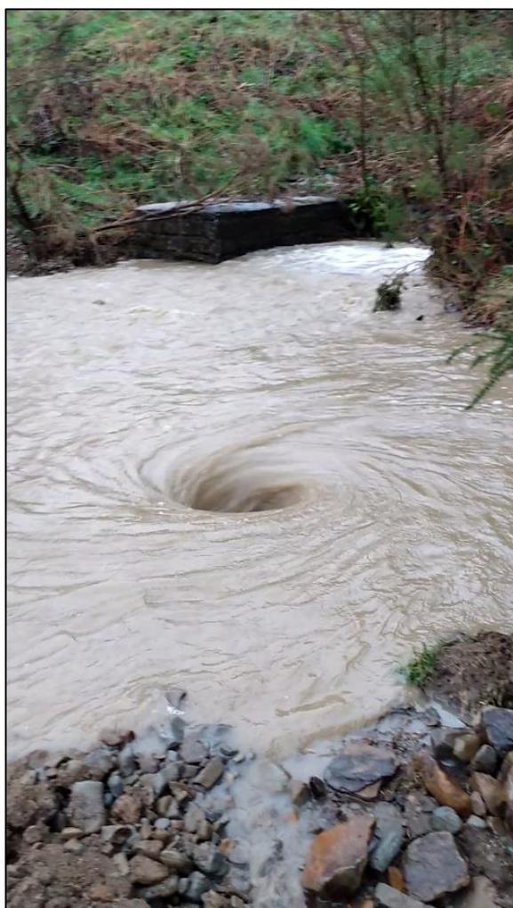
**Figure 6:** Whirlpool above the fully submerged 'Culvert Inlet 2' during Storm Dennis (image provided by resident)
