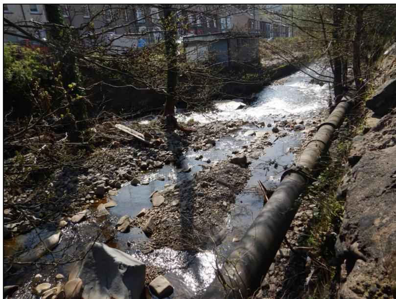
**Figure 20:** Debris accumulation along the channel bed of the Rhondda Fach River upstream of the footbridge between Standard View and Springfield Estate (image captured by RCTs Infrastructure team on 17<sup>th</sup> February 2020)
