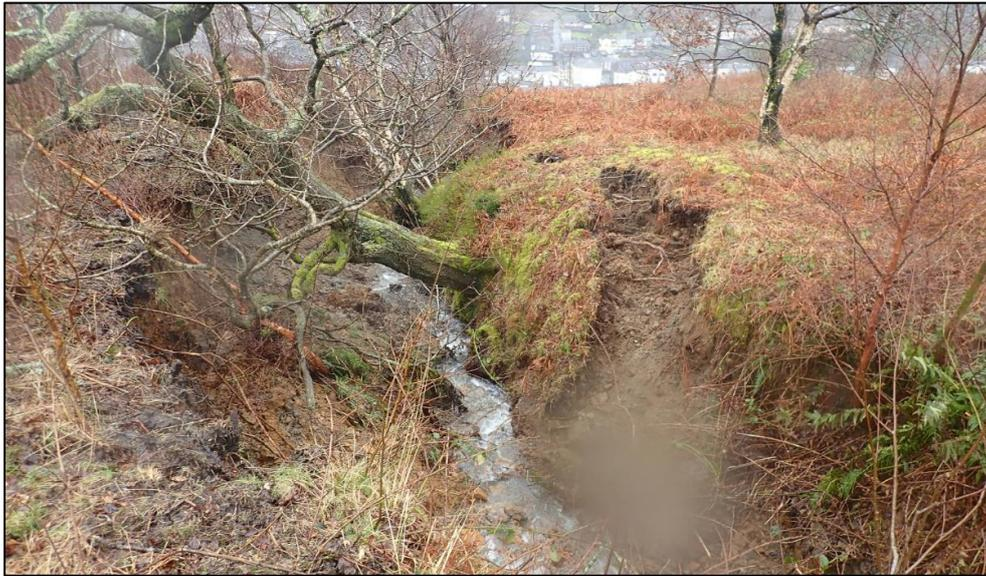
**Figure 15:** Evidence of eroded embankments within the ordinary watercourse upstream of 'Culvert Inlet 1' (captured by RCT's Flood Risk Management team on 19/02/2020)
