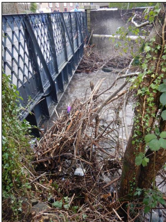
**Figure 9:** Image capturing accumulated woody debris on the embankment of the Rhondda Fach River behind the highway bridge following Storm Dennis (Image captured by a RCT Structures officer on 17<sup>th</sup> February 2020)
