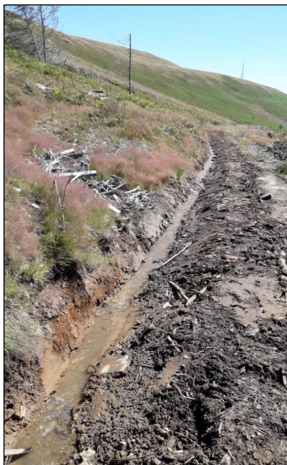
Figure 7: Image of the undefined ordinary watercourse / land drainage channel on the topside track above Aberdare Road following excavation works carried out by NRW in August 2020
