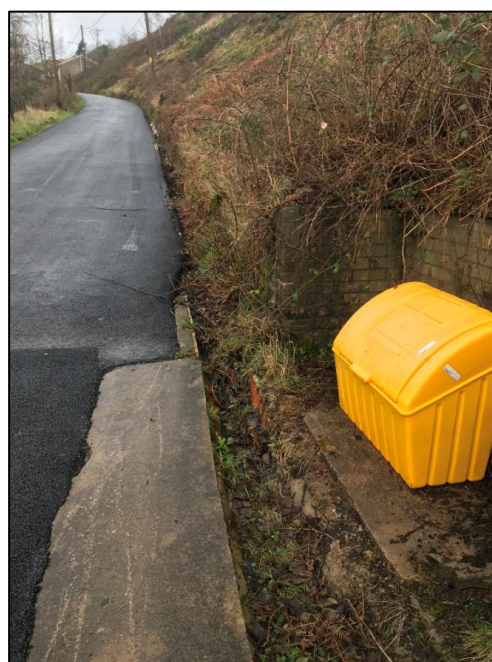
Figure 11: Condition of the highway drainage channel adjacent to Aberdare Road (captured by RCT's Flood Risk Management team on 18 th February 2020)
