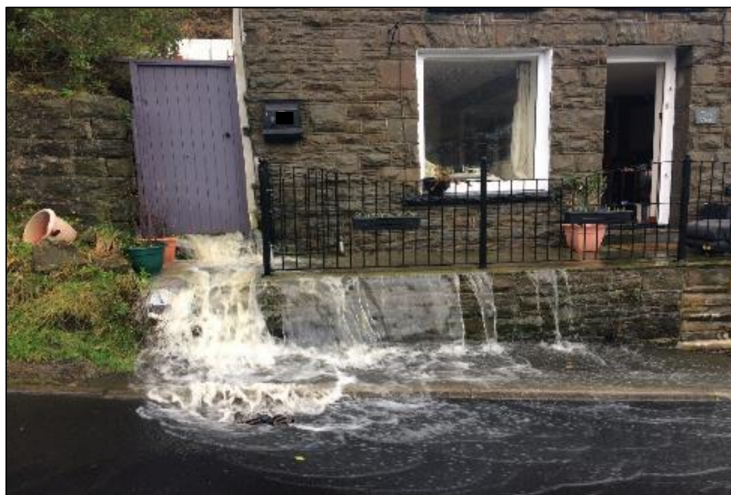
Figure 3: Pathway of flooding conveying from the side of a property at Aberdare Road and flowing down the steep road during Storm Dennis (image provided by resident)
