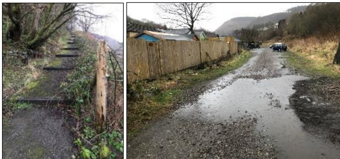
Figure 4: Post Event: Steps and path to the rear of Taff Street that the water flowed down during the event (left) and surface water pooling on the lane to the rear of Taff Street (right)
