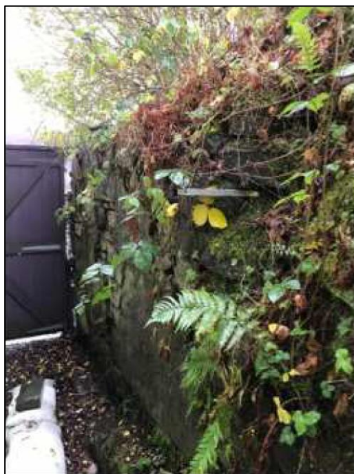
Figure 12: Photograph showing visual condition of the 'Retaining Wall 2' adjacent to a property at Aberdare Road
