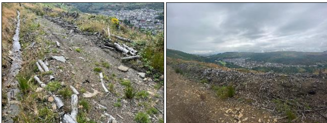
Figure 8: Evidence of woody material piled on the eastern side of the forestry access road, acting as an embankment (captured by RCT officers post NRW clearance works)
