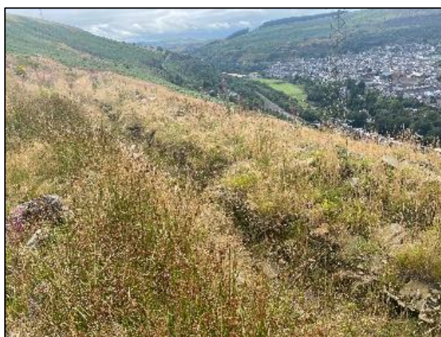
Figure 9: Drainage ditch identified below the forestry access road upon RCT's site visit
