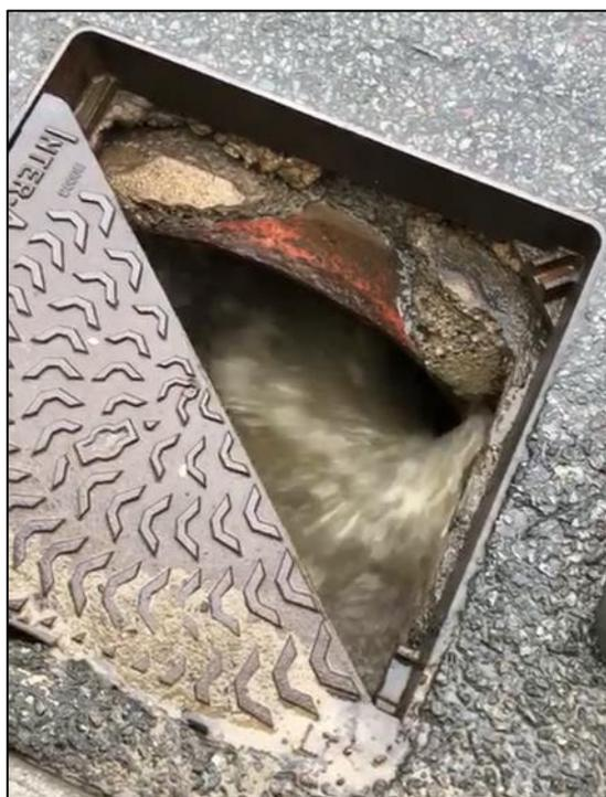
**Figure 10:** Photo of 'Manhole 1' surcharging during Storm Jorge (captured by RCT's Flood Risk Management team on 28<sup>th</sup> February 2020)
