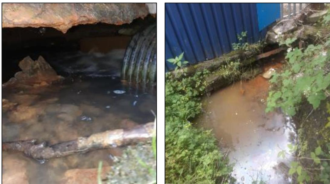
**Figure 13:** Outfall pipe entering 'Culvert Inlet 2' (left) and standing water surrounding 'Culvert Inlet 2' (right) (captured during CCTV survey operations on 30/06/2020)
