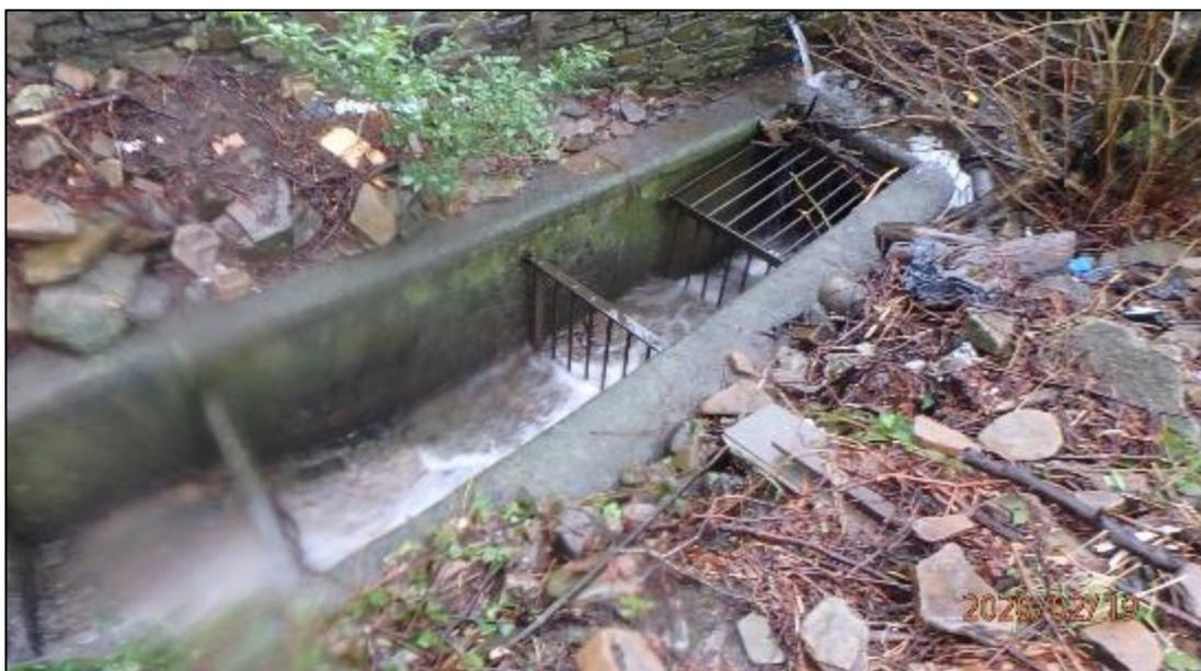
**Figure 7:** 'Culvert Inlet 3' to the rear of Dumfries Street which surcharged during Storm Dennis (captured by RCT's Flood Risk Management team on 19<sup>th</sup> February 2021)
