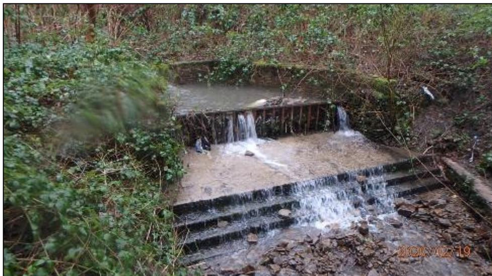
**Figure 22:** Photo of debris deposition behind the upper debris screen of the Nant Coedcaetylefforest ordinary watercourse (captured by RCT's Flood Risk Management team on 19/02/2020)
