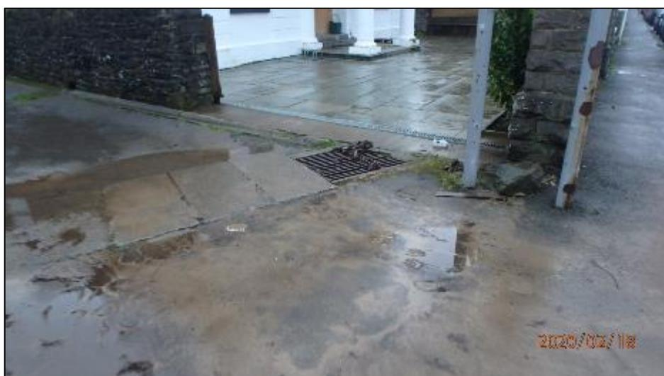
**Figure 6:** 'Manhole 1' located at Abertonllwyd Street surcharged during Storm Dennis (captured by RCT's Flood Risk Management team on 18<sup>th</sup> February 2021)
