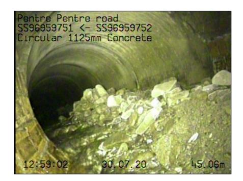
Figure 20: CCTV survey footage showing stone deposits between nodes SS96959751 and SS96959752 of the Pentre Road culvert network
