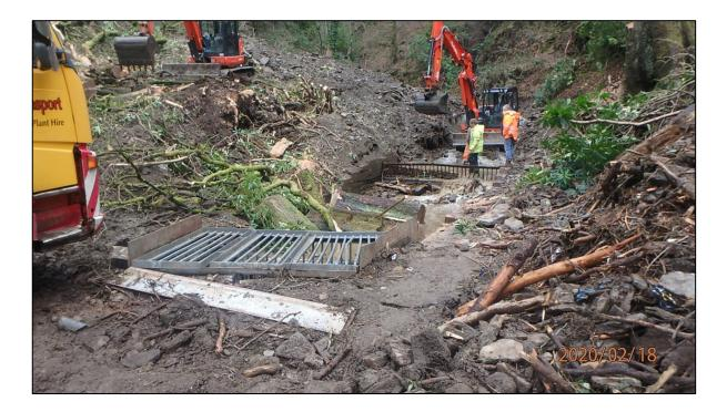
Photo provided by RCT's Flood Risk Management team of the Pentre Road culvert inlet and channel following emergency clearing works on 18<sup>th</sup> February 2020.
