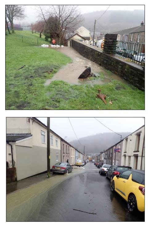
**Figure 9**: Surcharging manhole within Pleasant Street Park (top) and flow path down Pleasant Street (bottom) taken by RCT's FRM team on 20<sup>th</sup> February 2020
