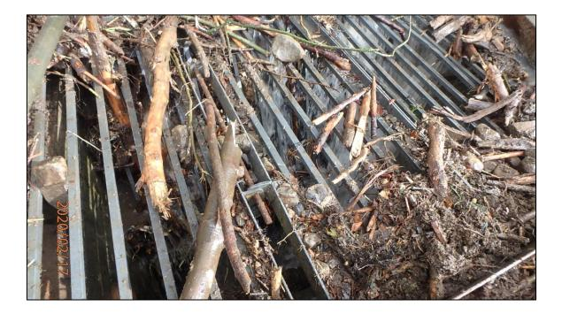
Photo provided by RCT's Flood Risk Management team showing woody debris in the Nant y Pentre channel and at the culvert inlet on 17<sup>th</sup> February 2020.
