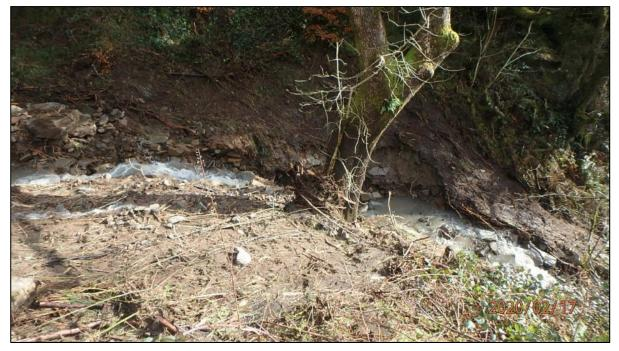
Figure 23: Photo of minor scour to the embankments of the Nant y Pentre watercourse in the upper catchment of Pentre (17/02/2020)
