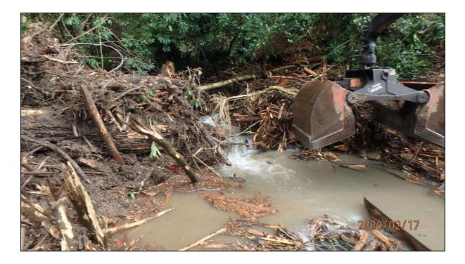
Photo provided by RCT's Flood Risk Management team showing woody debris on the debris screen of the Pentre Road culvert inlet on the 17<sup>th</sup> February 20020.
