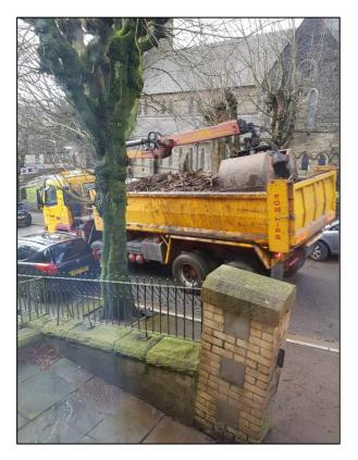
Figure 18: Photo showing woody debris being transported away from the Pentre Road culvert inlet during emergency clearance works (17/02/2020) (image provided by resident)
