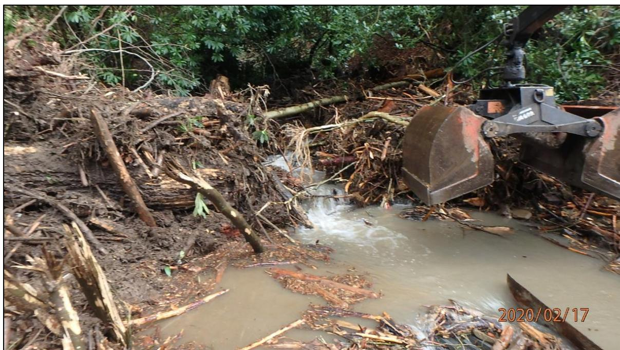
Photo provided by RCT's Flood Risk Management team showing woody debris on the debris screen of the Pentre Road culvert inlet on the 17<sup>th</sup> February 2020.
