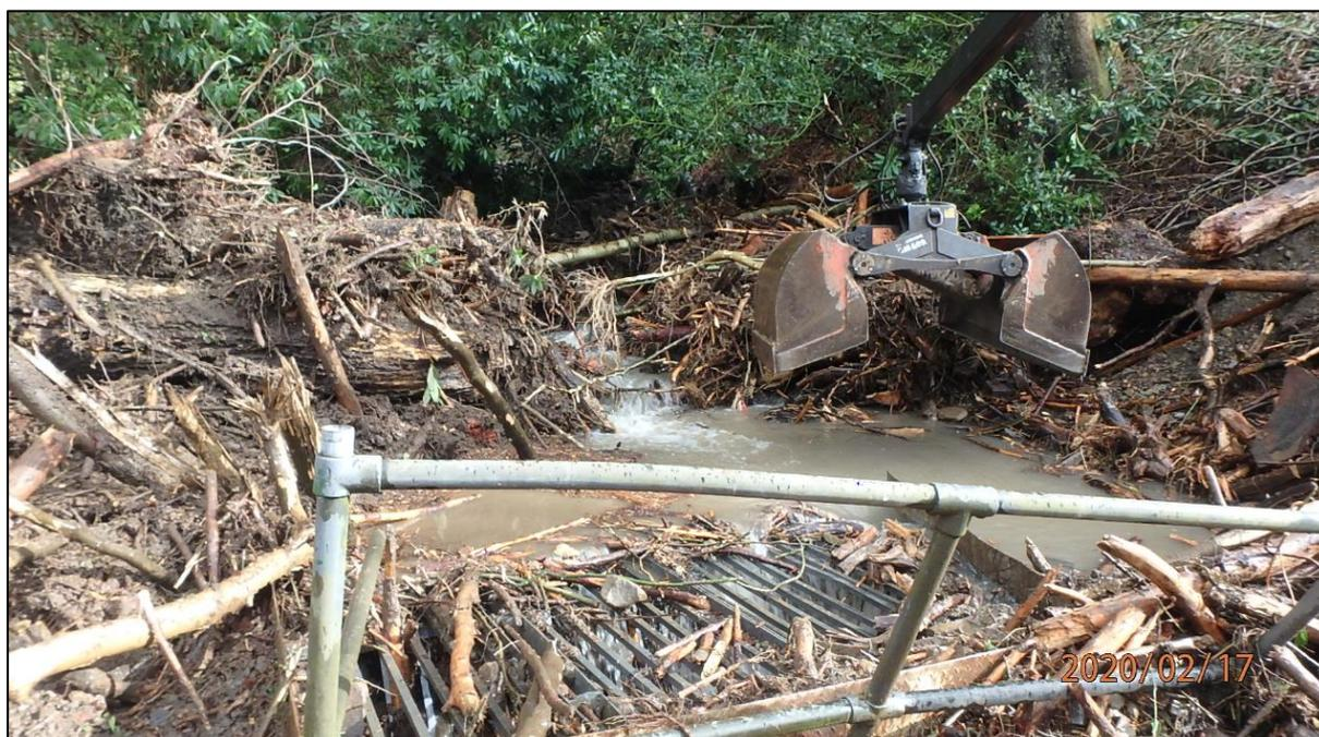
**Figure 15:** Photo of Pentre Road culvert inlet during works to remove deposited material post Storm Dennis (17/02/2020)
