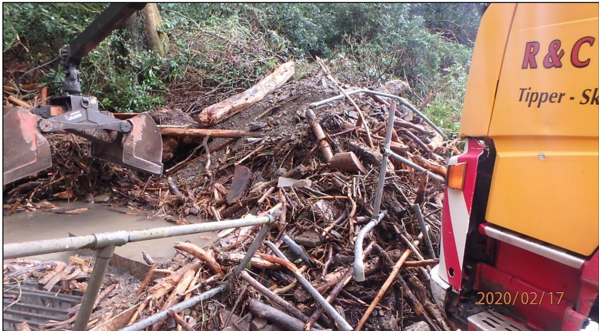
**Figure 16:** Photo looking across the Pentre Road culvert inlet, showing significant material collected during Storm Dennis (17/02/2020)
