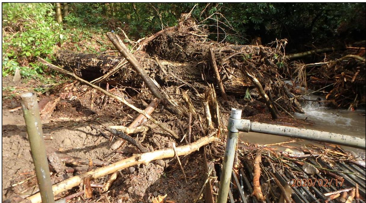
**Figure 17:** Photo of Pentre Road culvert inlet showing significant woody debris deposition (17/02/2020)
