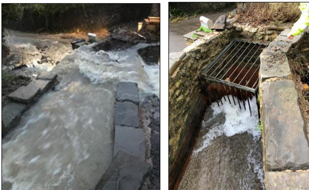
**Figure 5:** Evidence of 'Culvert Inlet 1' surcharging during the storm event and conveying southwards towards Column and Dumfries Streets (left) (image provided by resident), and 'Culvert Inlet 1' post storm event (right) (captured by RCT's Flood Risk Management team on 20<sup>th</sup> February 2020)
