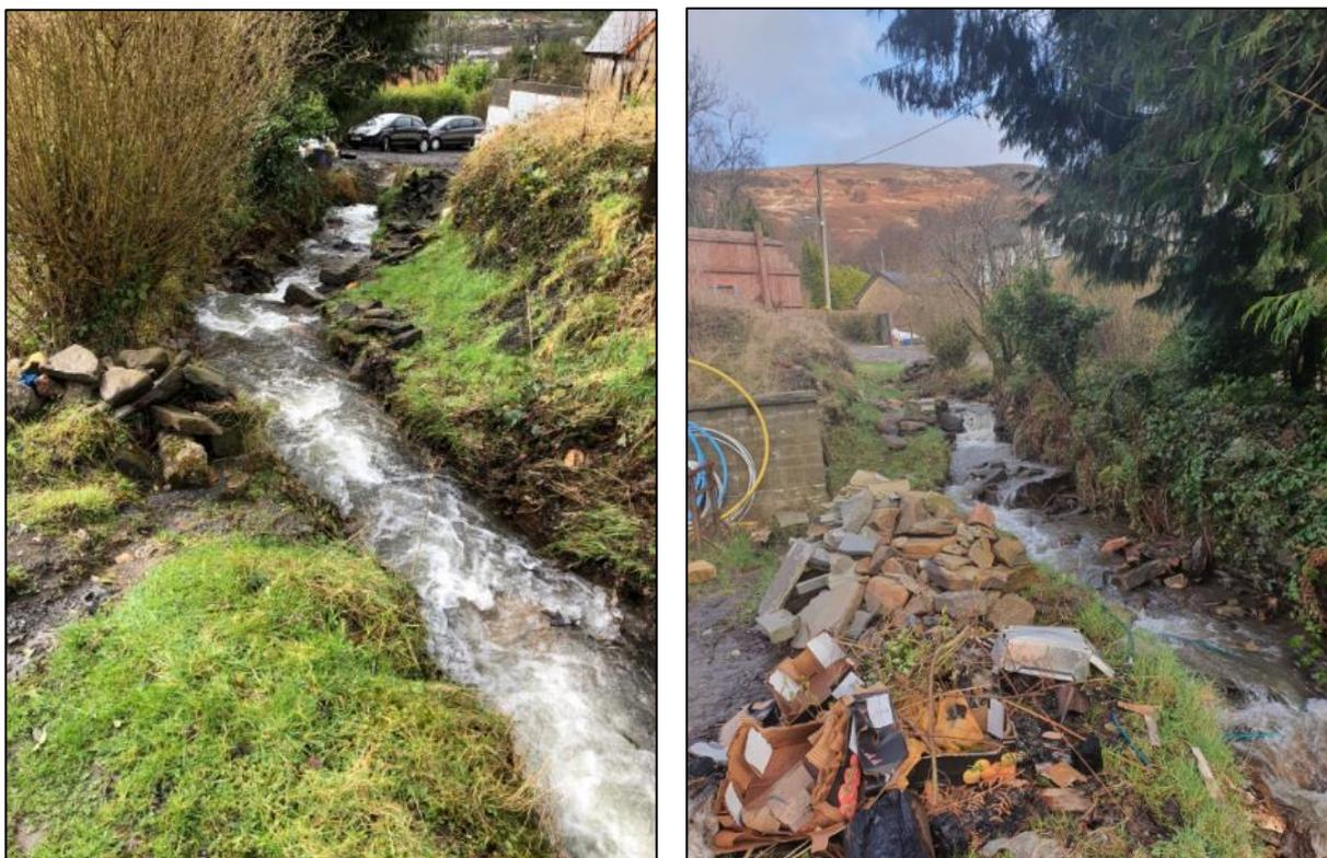
**Figure 22:** Unnamed open watercourse upstream of 'Culvert Inlet 1' showing evidence of large stones within the channel and surrounding embankment area (captured by RCT's Flood Risk Management team on 20<sup>th</sup> February 2020). Looking downstream towards 'Culvert Inlet 1' (left) and looking upstream towards the outfall of 'Culvert Inlet 2' (right).
