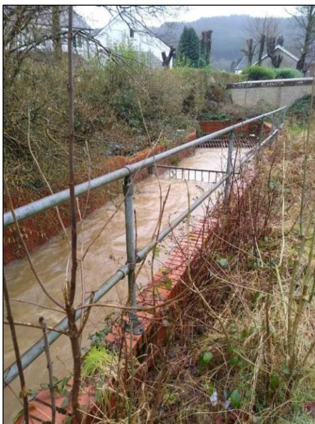
**Figure 16:** Column Street open channel and culvert inlet showing high flows (image provided by resident. Captured at 11am on 16th February 2020)
