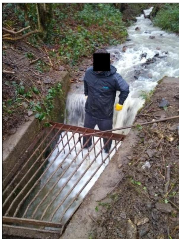
**Figure 15:** Photo of 'Culvert Inlet 3' following initial debris clearance by local residents on 16<sup>th</sup> February 2020.
