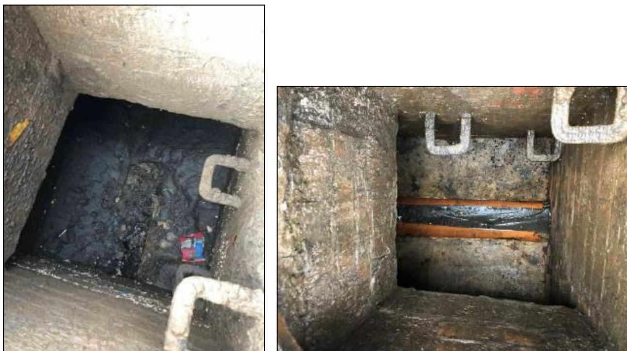
**Figure 17:** Photo of a manhole at Fountain Street captured before (left) and after (right) surveying and cleansing operations during April 2020
