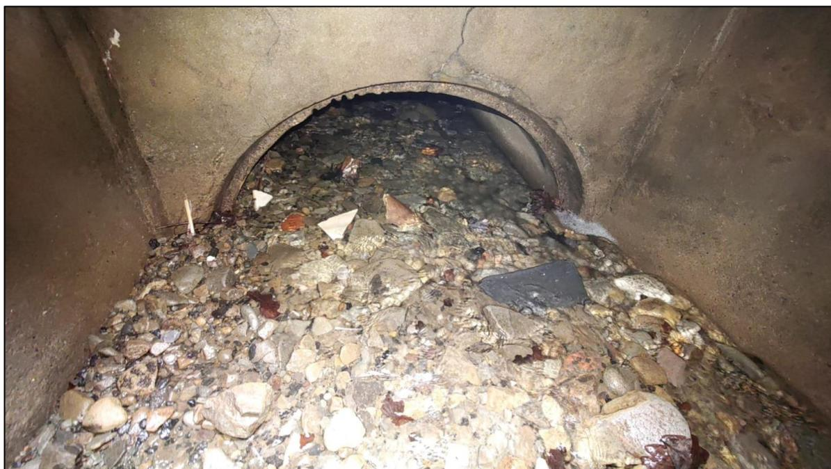
**Figure 14:** Debris accumulation within the culvert network downstream of 'Culvert Inlet 1' (view looking upstream from Manhole 1) captured post event during CCTV surveying operations
