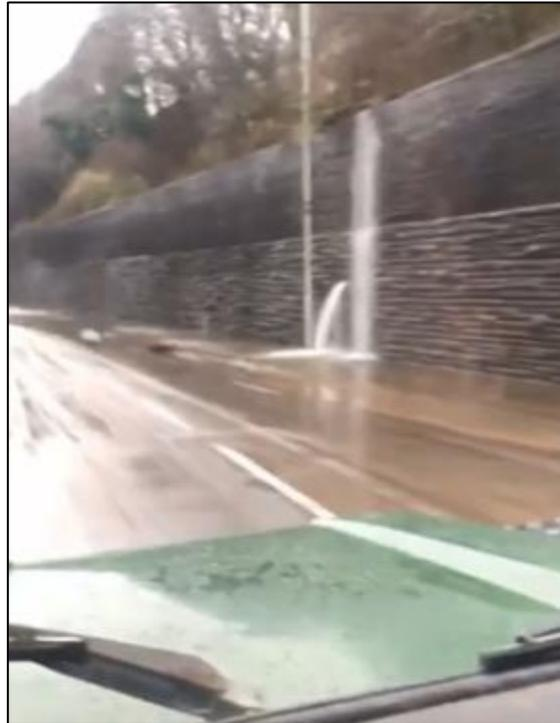
**Figure 6:** Image capturing water overtopping and breaching through the retaining wall below 'Culvert Inlet 1' and the A4058 during Storm Dennis (Source: Social Media)
