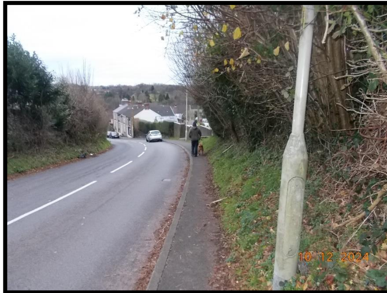
Photograph 4.5 – Leaf debris causing localised footway narrowing on Cardiff Road, where pedestrians are required to step into the road to pass one another
