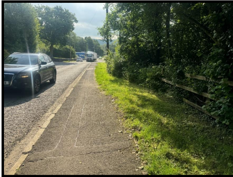
Photograph 4.23 - Localised footway narrowing with vegetation encroachment on the B4278
