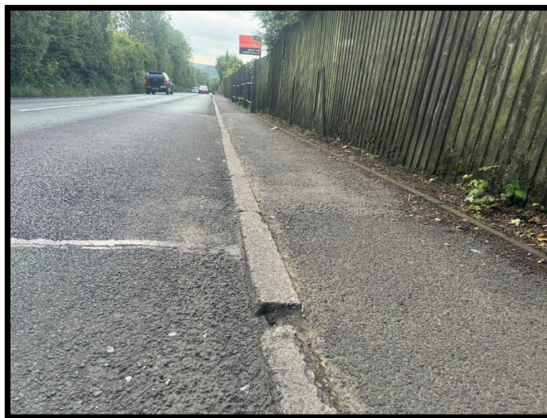
Photograph 4.21 - Eastern footway flush kerbs on A4093 (40mph) and footway narrowing to circa 1.0m
