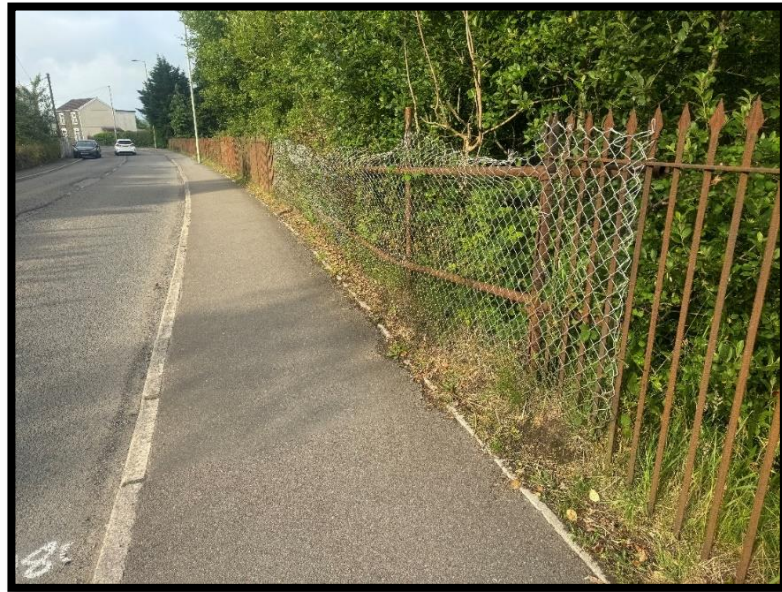
Photograph 4.3 – Overhanging chain-link fence western footway B4564
