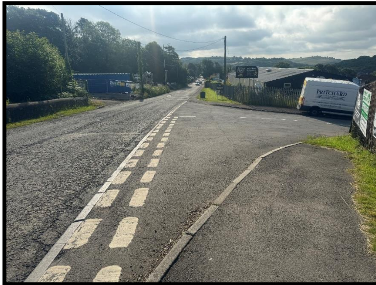
Photograph 4.24 – Reduced visibility issues at uncontrolled crossing point on the junction of the fencing supplier's unit and Gilfach Road, it is noted however that traffic flows are very low entering the unit
