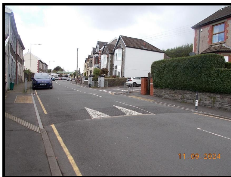
Photograph 4.1 – Uncontrolled raised crossing (road hump) at the junction access to Porth Community school
