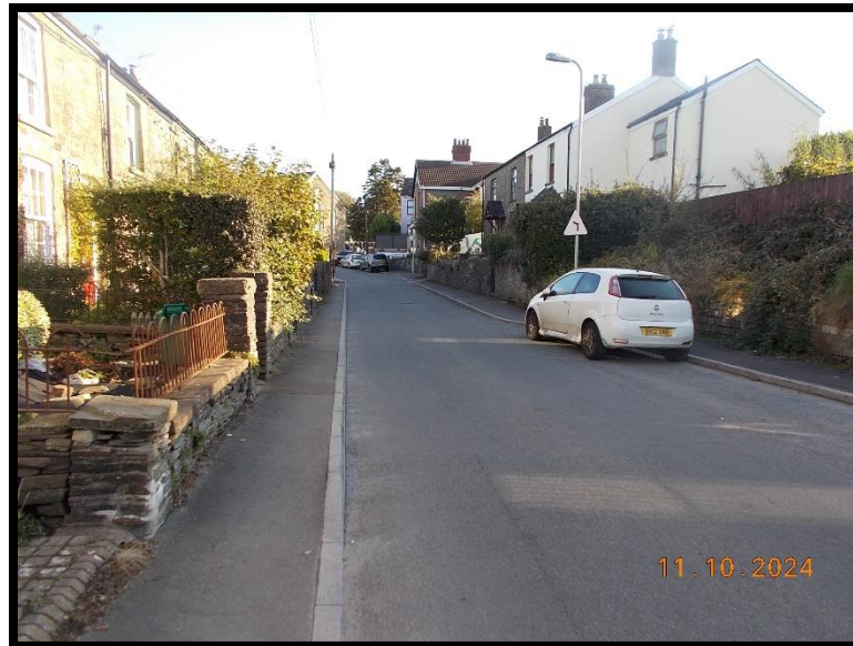
Photograph 4.36 – Narrow footways along Ffordd-Y-Capel at circa <1.0m width. This road was noted to have low vehicle and pedestrian flows during the time of the assessment
