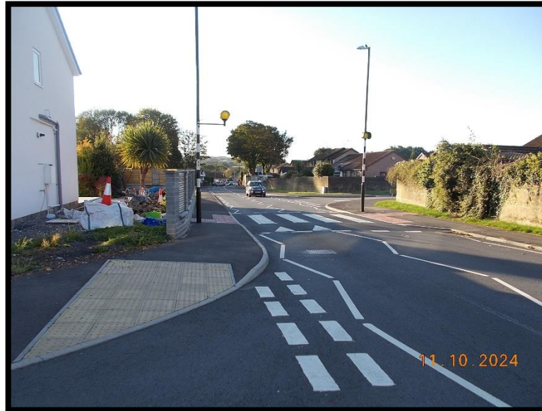
Photograph 4.43 – Raised Zebra crossing (road hump) near the junction of Aspen Way with Crown Hill
