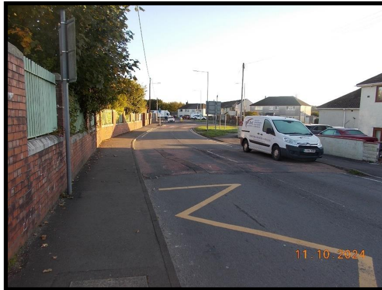
Photograph 4.28 – Uncontrolled crossing link over the existing speed hump (near the school exit) obstructed by on-street parking
