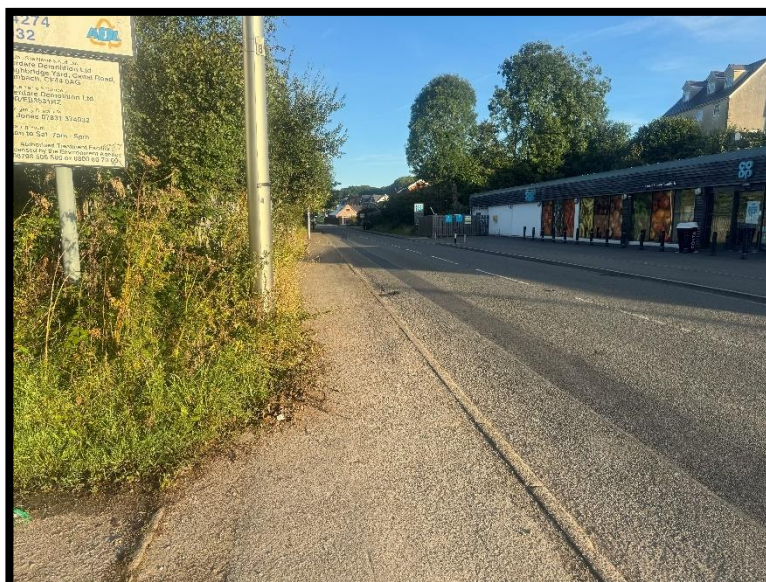
Photograph 4.7 – Overgrown vegetation on western footpath of Canal Road reducing the usable width
