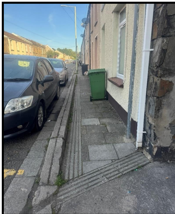
Photograph 4.19 – Back-to-back kerbs with refuse wheelie bins reducing usable footway along Gloucester Street
