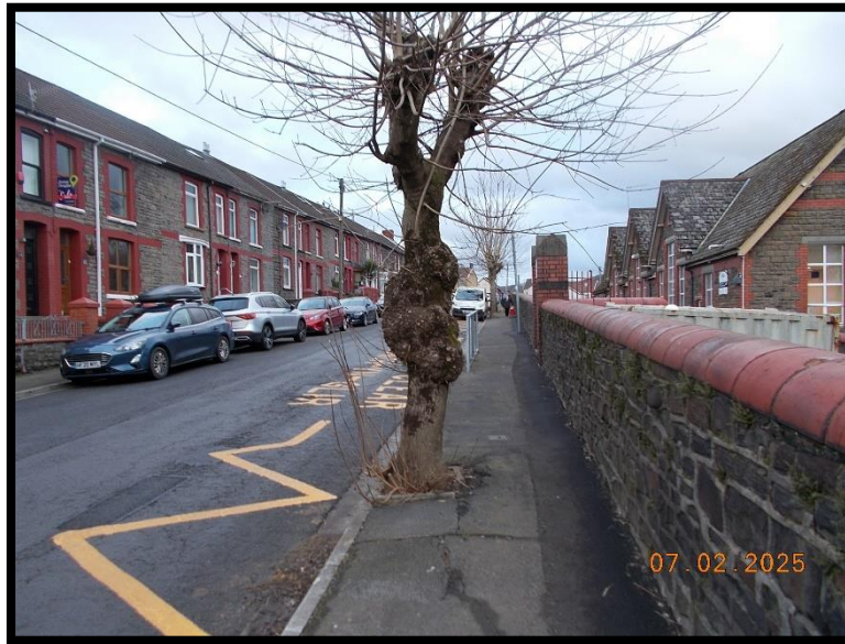
Photograph 4.23 – Localised footway narrowing with uneven footway profile due to tree planting outside Maes Y Coed Primary School
