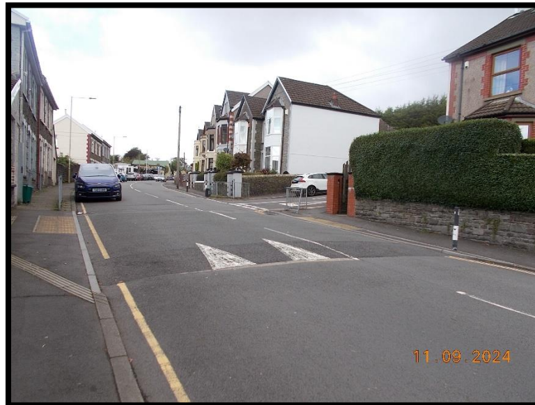
Photographs 4.25 – Uncontrolled raised crossing on the B4278 Cemetery Road near the entrance to Porth Community School
