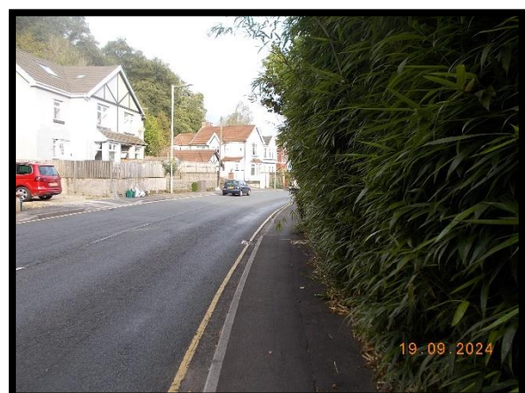
Photograph 4.30 & 4.31 – Overhanging vegetation narrowing the usable footway width along the B4595 Llantwit Road
