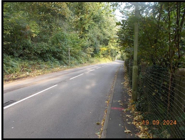
Photograph 4.32 – Localised footway narrowing at lighting columns and overhanging vegetation along the B4595 Llantwit Road within the 40mph speed limit
