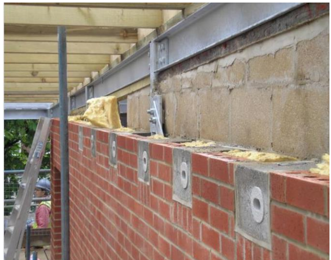
Swift bricks in wall of a house being built
