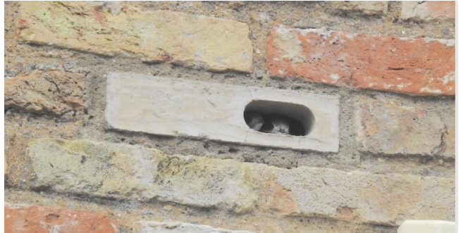
"S-Brick" in wall of a house made by Action for Swifts (Dick Newell).
