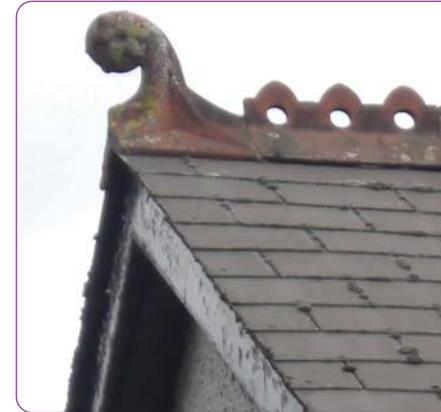
*Where there is no chimney, a scrolled finial forms a punctuation to the gable end.*
