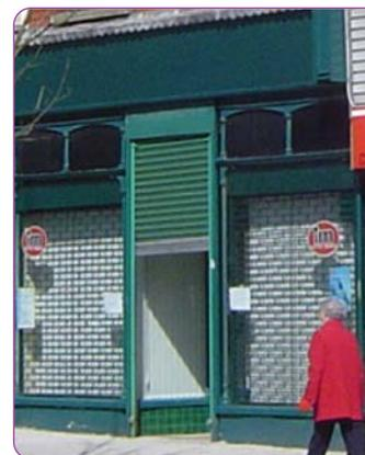
*A lattice brick shutter (preferably internal) provides a much more subtle feature than a bulky solid roller shutter.*
