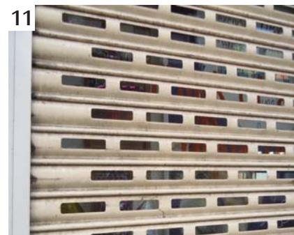
If alternatives are clearly demonstrated not to be appropriate, external metal roller shutters may be considered, depending on the type and location of the building. **However, solid metal roller shutters are unlikely to be considered acceptable (6).**
